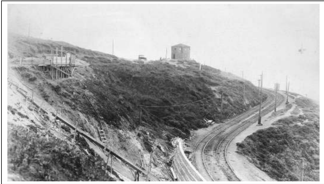
Figure 30. Construction work on El Camino Del Mar in June 1923. One of the two retaining walls constructed by the city's DPW to protect the streetcar tracks is visible at lower right. The large building is the Marine Lookout on the future site of the USS San Francisco Memorial. (SF Public Library, DPW)
