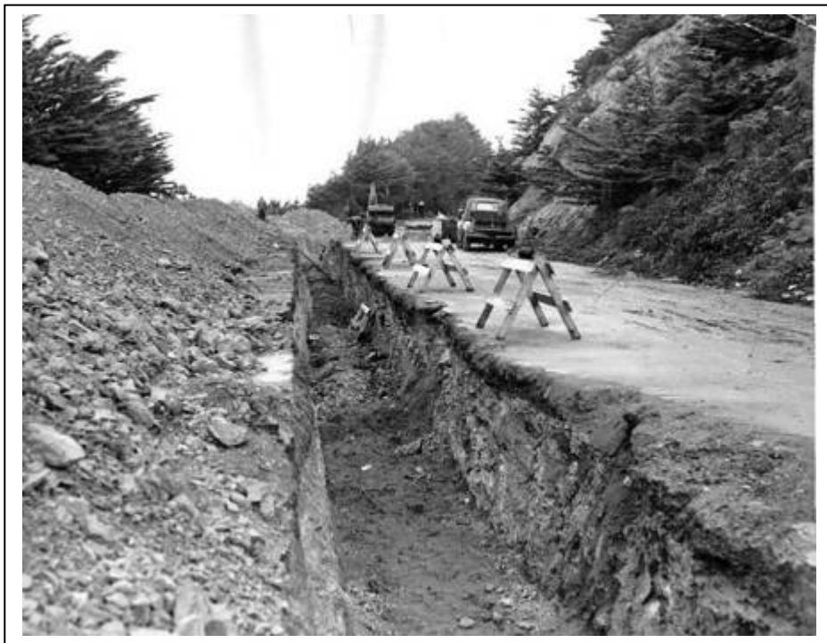
Figure 75. El Camino Del Mar drainage ditch construction, November 15, 1957 (SF Public Library AAB-9169)
