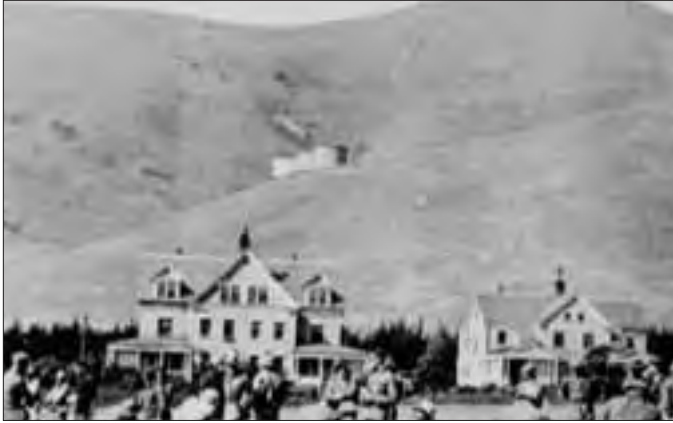
NS2 Water was pumped to storage tanks located on the hills above the cantonment. The hills provided a head to build water pressure to supply Fort Baker. Circa 1915 (GGNRA Park Archives and Record Center, 3311.007).
