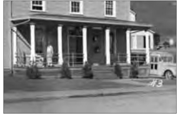
Sidewalk Curb, Circa 1938 Location: FB603 Extant
