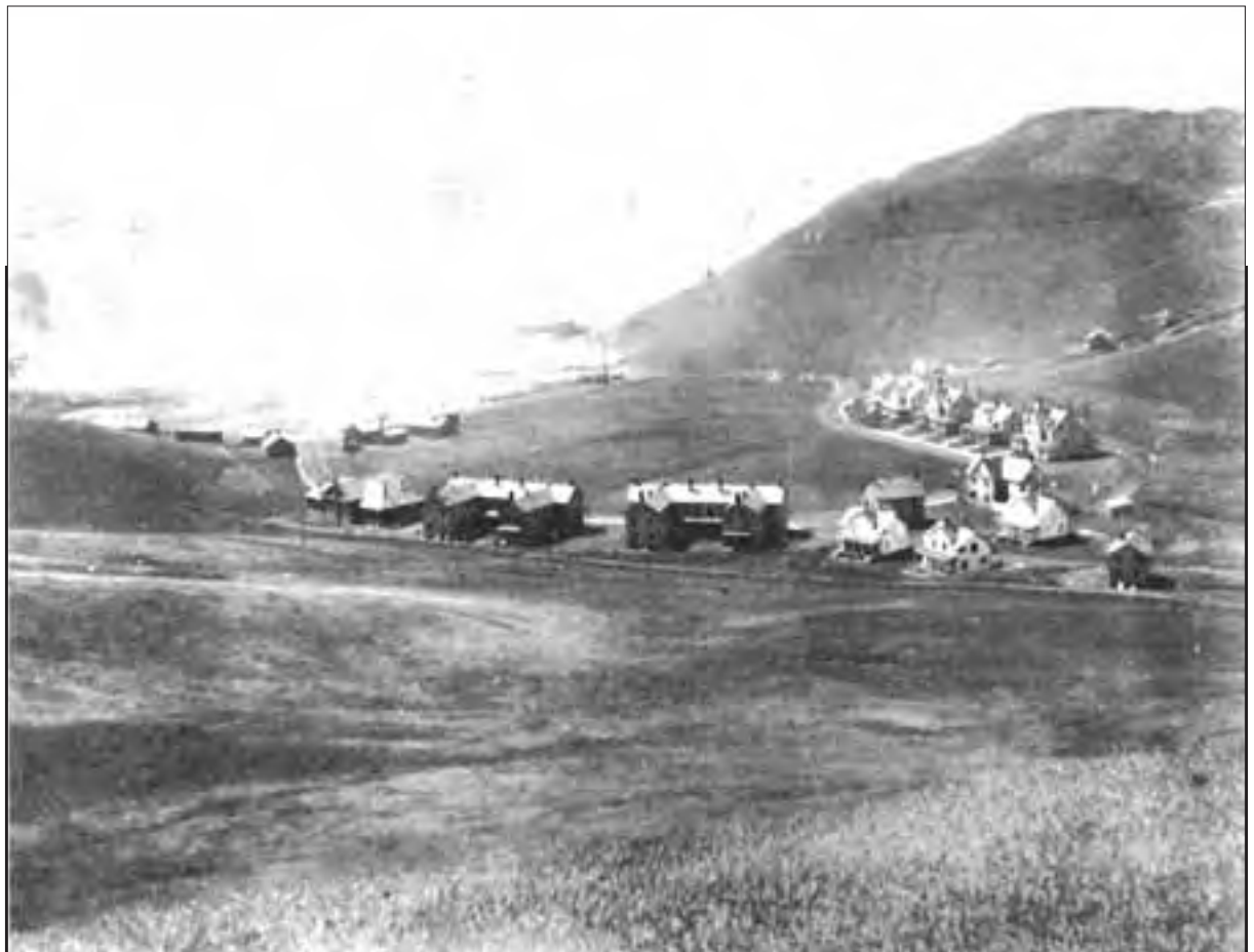
NS3 The valley north of Horseshoe Cove was a relatively flat and natural setting for buildings, a microclimate buffering the cantonment from inclement weather. Circa 1904-6 (Sausalito Historical Society, Chambers Family Photo Collection, Negative 9846.3).
