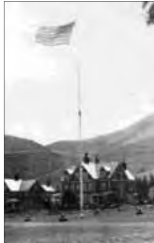
Flagpole, Circa 1915 Location: Parade Ground, looking northwest Flagpole: Extant Compass Rose treatment: Removed
