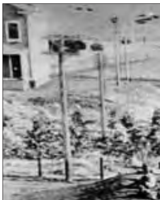
Utility Pole, Circa 1915 Location: East side of Murray Circle, (FB601) looking east Extant
