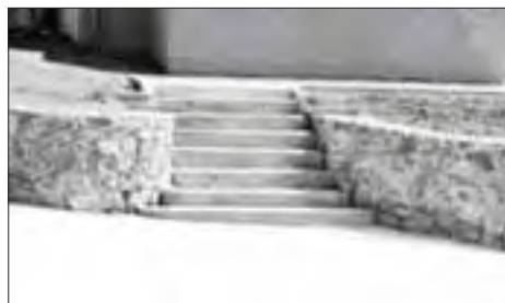
Stairs 4 and Stone Retaining Wall, Circa 1938 Location: FB527 Extant
