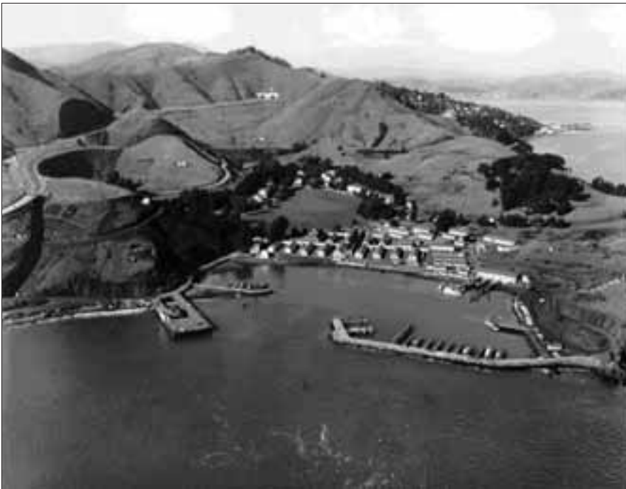
SH17 Mine depot structures clustered near the waterfront included storehouses, cable tank building and powerhouse, looking northeast. Circa 1941 (GGNRA Park Archives and Record Center, 2266-N1,02).
