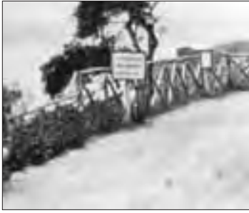
Fence, Circa 1900 Location: East Road Entrance Removed
