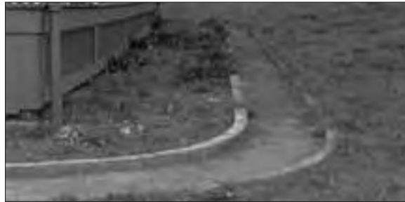
Walkway, 2001 Location: FB607 Extant
