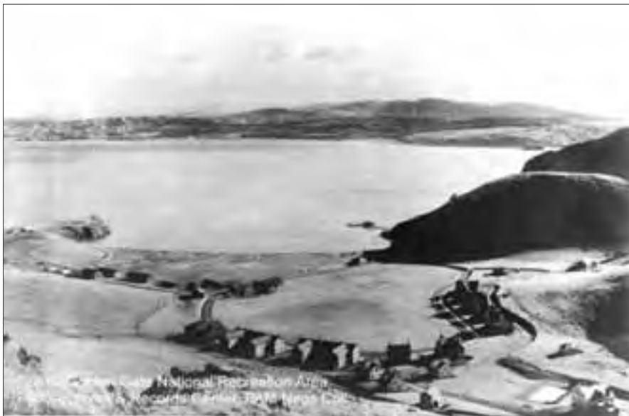
SH4 Parade ground and Murray Circle. Note extent of cut required for construction of the parade ground and preparation of building site. Looking south. Circa 1905 (GGNRA Park Archives and Record Center, 40039.014).
