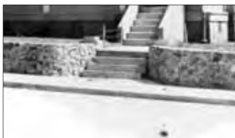
Stairs 3 and Stone Retaining Wall, Circa 1938 Location: FB523 Extant
