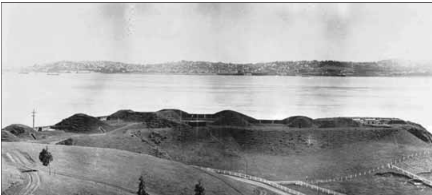
T1 The silhouette of Cavallo Battery against the San Francisco Bay illustrates the extensive use of earth works in early battery construction. Circa 1914 (GGNRA Park Archives and Record Center, 1766).
