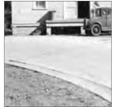
Road Gutter, Circa 1925 Location: FB631 Extant
