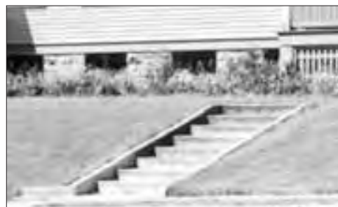
Stairs, Circa 1938 Location: FB631 Extant
