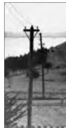
Utility Pole, Circa 1915 Location: West side of Murray Circle, looking south Extant
