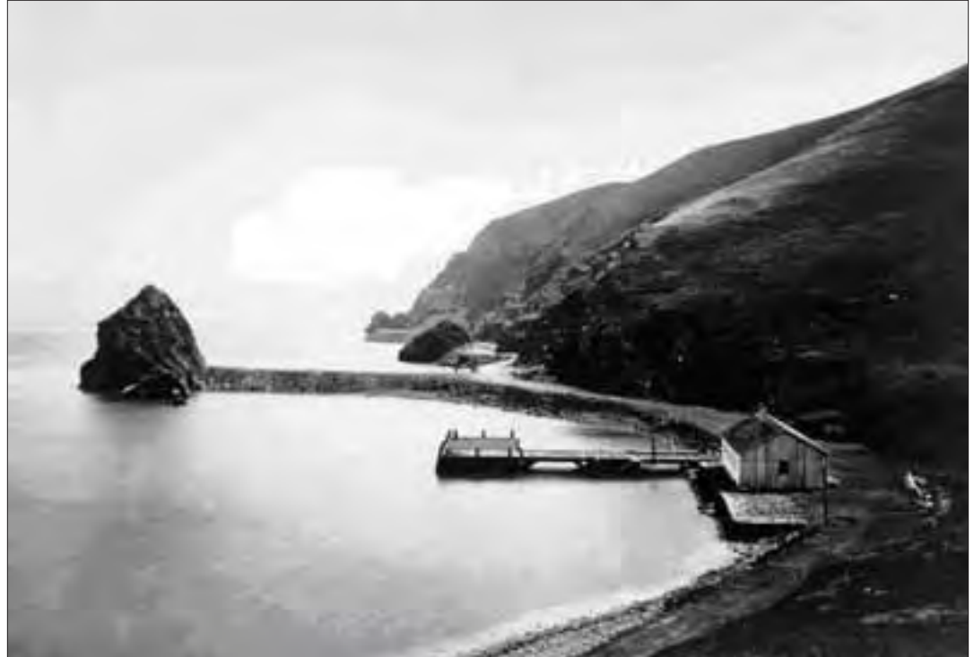
SH1 Engineer Wharf on lee side of Needles breakwater, near west end of Horseshoe Cove, looking west. 1868 (National Archives and Record Center, RG #77-F-100-140).
