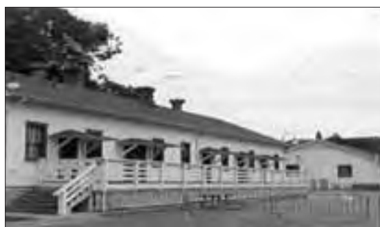
Railing, 2001 Location: Service area Extant
