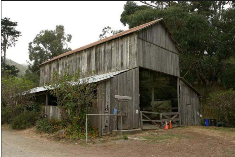
The original milking barn was destroyed by fire in the 1920s. This replacement was constructed during the period of significance, and is a contributing resource.
