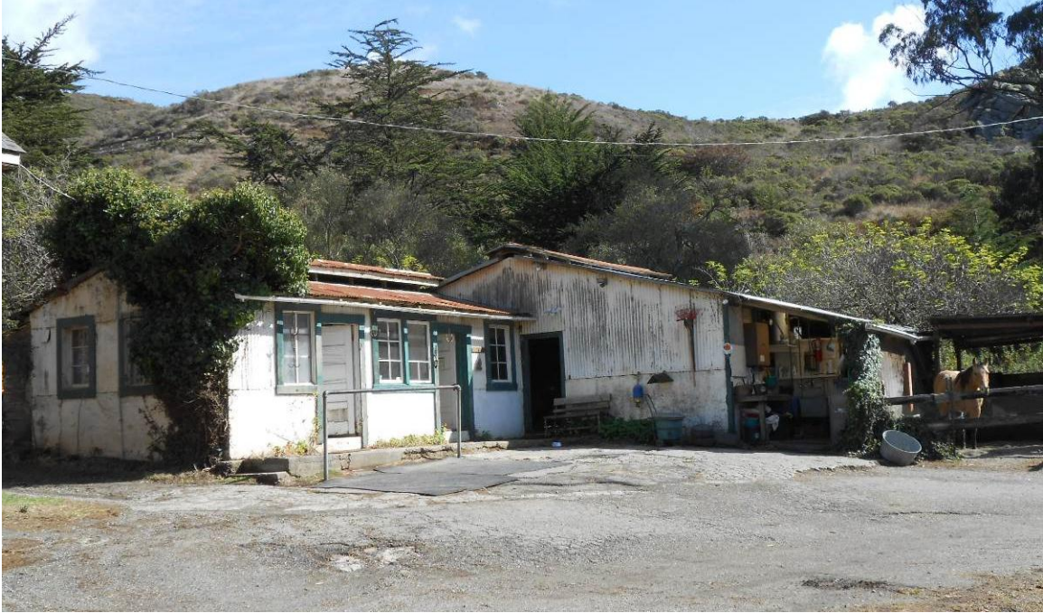
Sanitary Barn at the Golden Gate Dairy Looking Southeast (NPS Photo, 2010)
