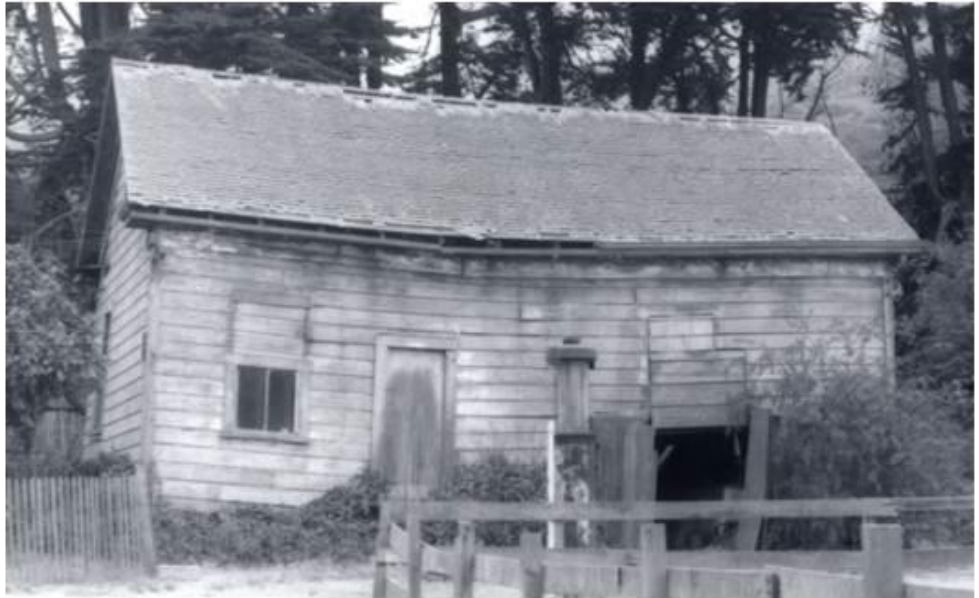
Golden Gate Dairy Creamery Building South Façade ca. 1970
