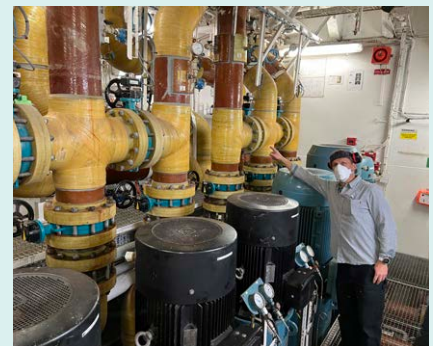
An NPS Scientist inspects the emission gas cleaning system ('scrubber') installed on a cruise ship operating in Glacier Bay.
