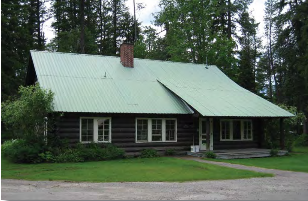
Figure 27. West Lakes District Office in 2011.
