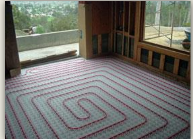
Example of In-Floor Radiant Heating
