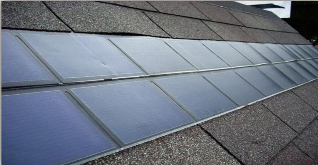
Example of PV Solar Shingles on Roof
