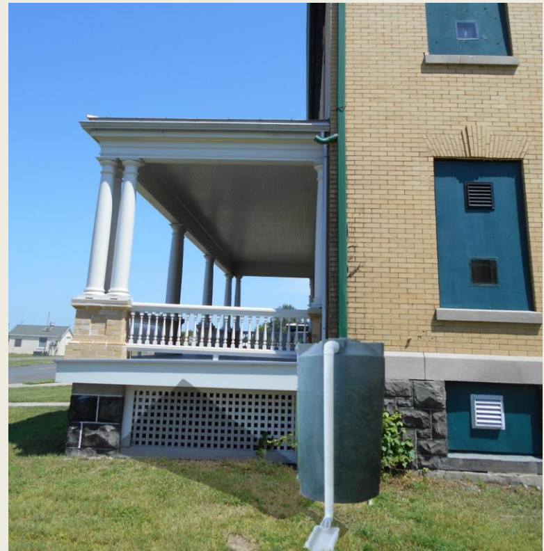
Example of Potential Rain Water Cistern at Building 7
