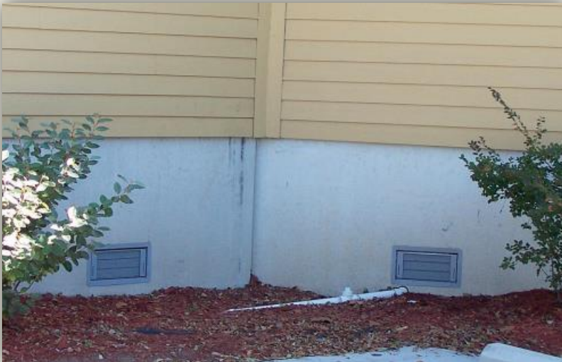
Example of Basement Flood Vents
