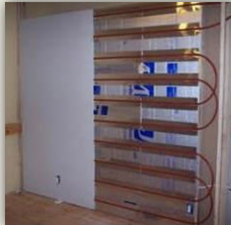
Example of PEX Wall Radiator
