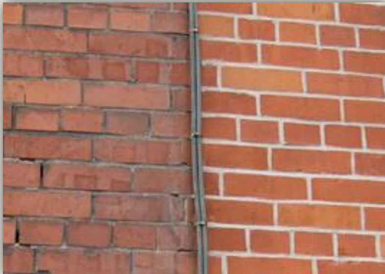
Example of Brick Repointing Before + After
