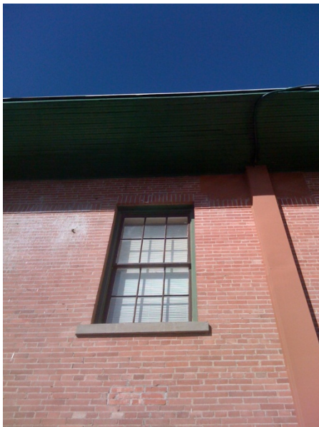
Building 115 – Window & Eave
