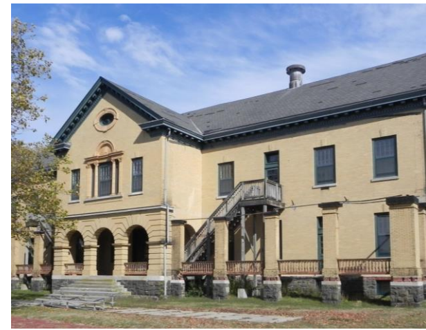
Buildings 24 (above) and 25 (below)
