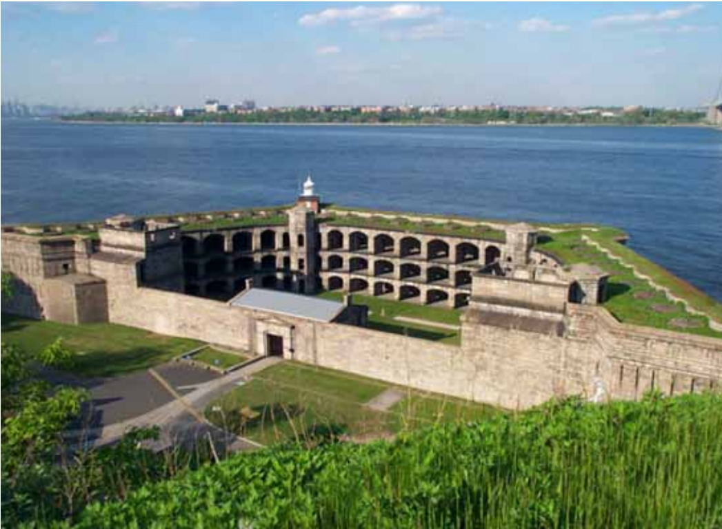
Figure 3-8. Battery Weed Looking Northeast Across the Narrows Toward Brooklyn (2006).
