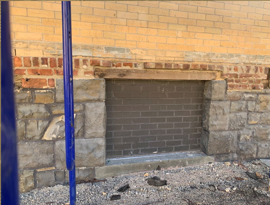
Building 56 – currently under construction
