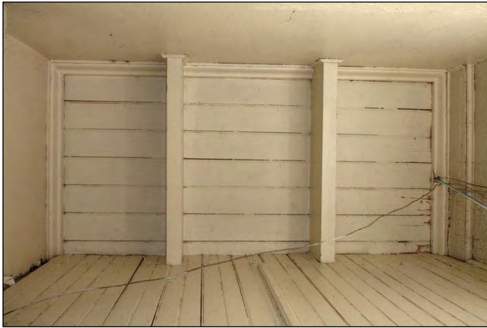
Figure 53. Spermaceti Cove Life-Saving Station, Room 104a ceiling.
