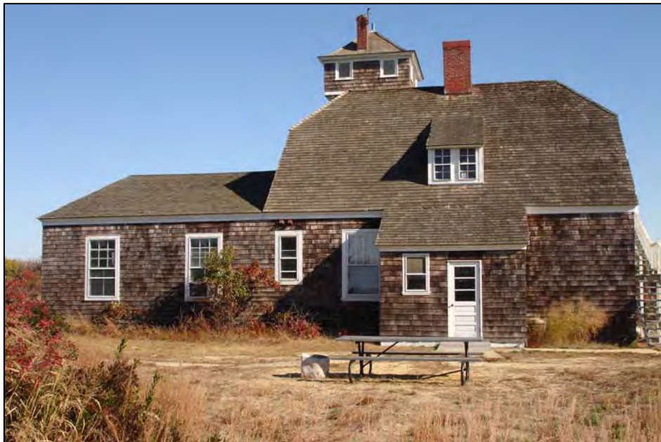
Figure 42. Spermaceti Cove Life-Saving Station, west elevation.
