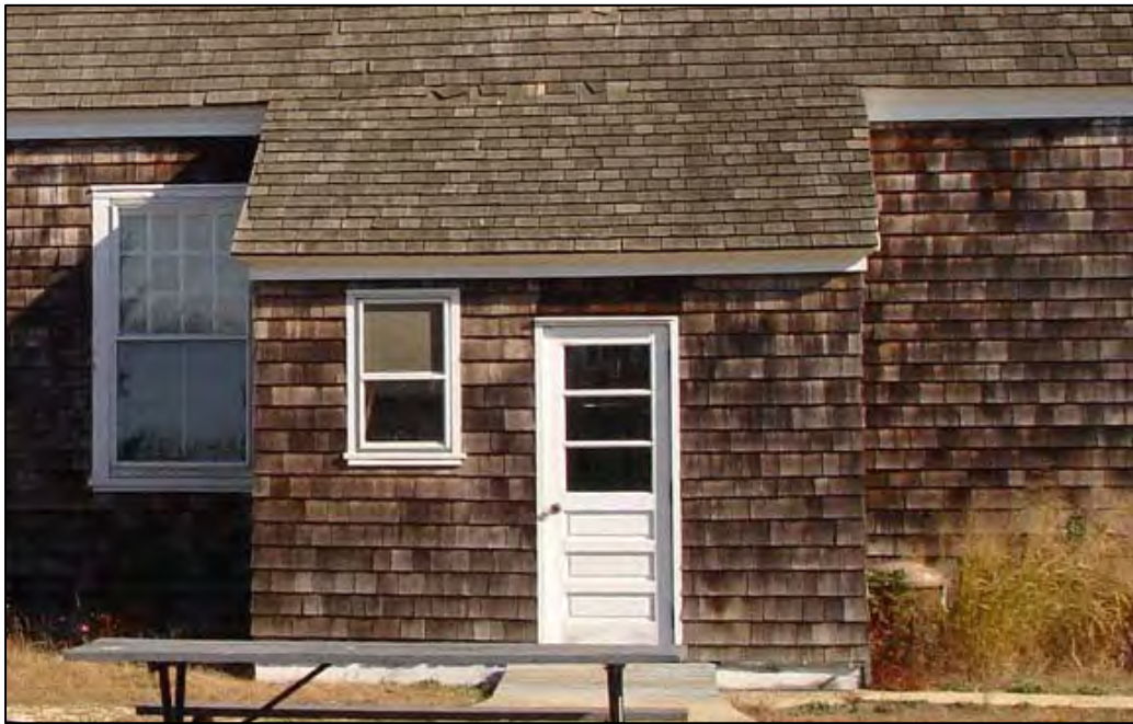
Figure 35. Spermaceti Cove Life-Saving Station, depicting west elevation exterior of enclosed back porch.
