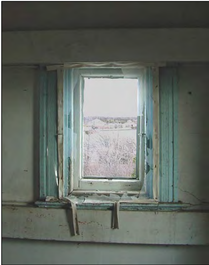
Figure 63. Spermaceti Cove Life-Saving Station, Room 301 W304 depicting window opening elements and alterations typical of third-story windows.
