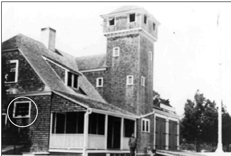
Figure 17. 1894 Spermaceti Cove Life-Saving Station, east and south elevations, circa 1916 depicting historic window openings including south elevation awning sash (circled). This photograph also depicts some post-1909 alterations to the station.
