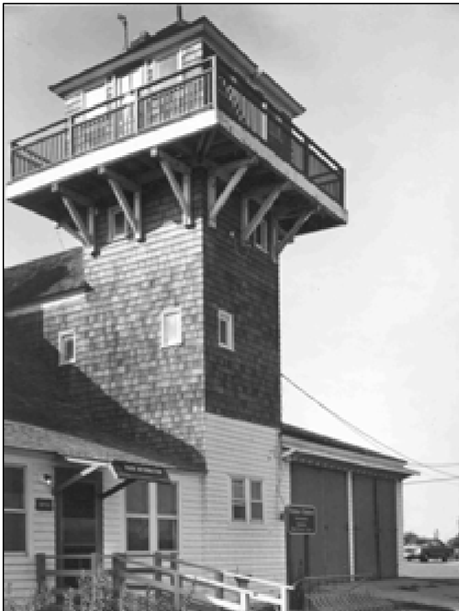
Figure 39. Spermaceti Cove Life-Saving Station, circa 1976 south and east elevations of Tower and connector after re-shingling of upper stories of Tower and roofs.
