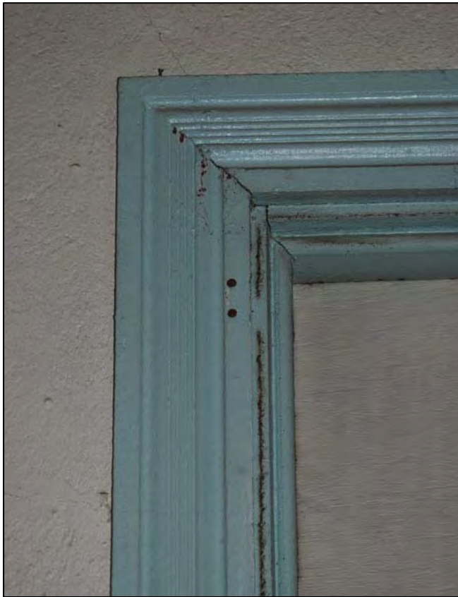
Figure 59. Spermaceti Cove Life-Saving Station, Room 205 W209 depicting window opening molded surround.
