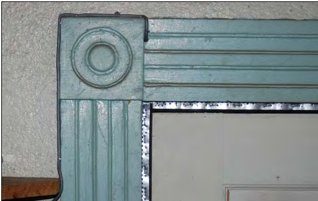
Figure 58. Spermaceti Cove Life-Saving Station, Room 205 D204 depicting doorway trim typical of interior doorway elements.
