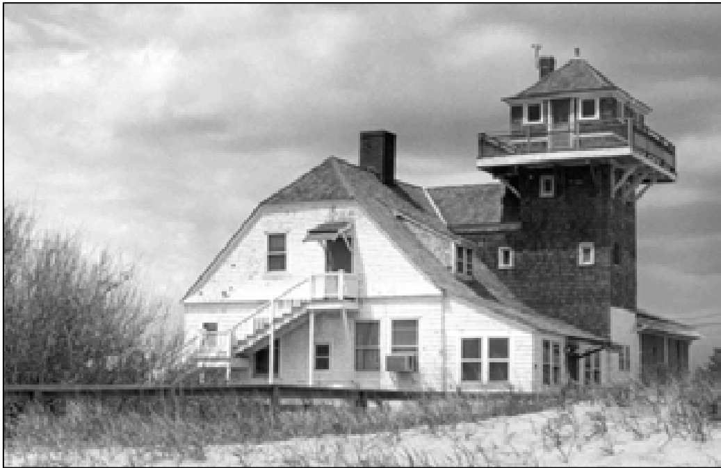
Figure 38. Spermaceti Cove Life-Saving Station, circa 1976, south and east elevations after re-shingling of Tower and roofs.
