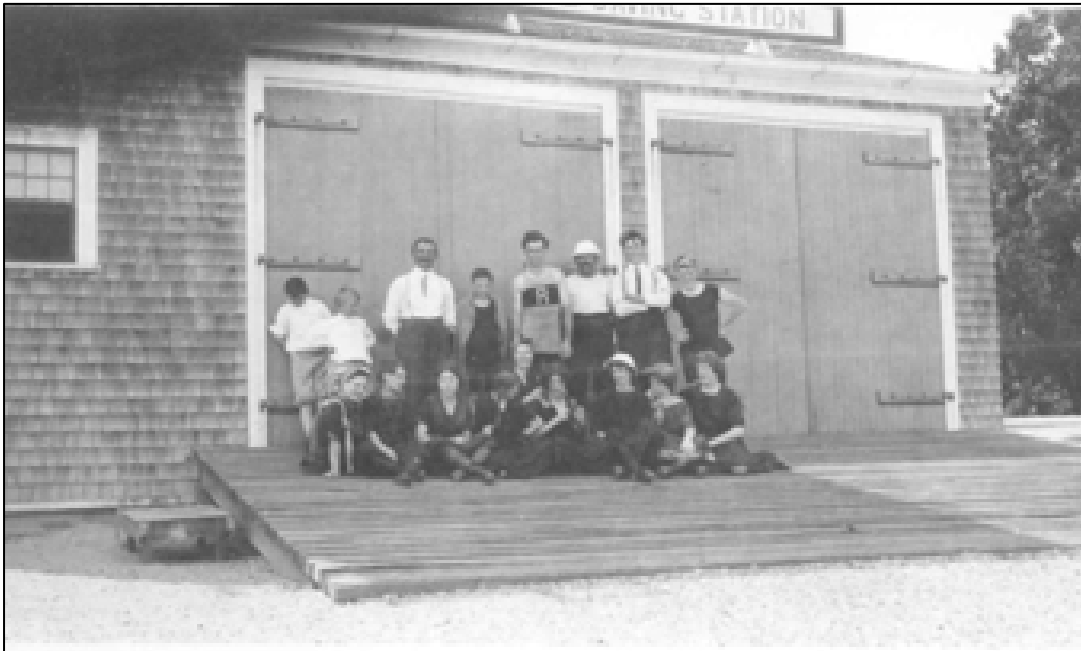
Figure 27. Spermaceti Cove Life-Saving Station, Capt. Joel Wolley and crew circa 1912, depicting east elevation post-1909 alterations to the Boat Room doorways.
