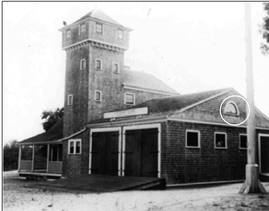
Figure 16. 1894 Spermaceti Cove Life-Saving Station, east and north elevations, circa 1916, depicting historic window openings including north elevation fanlight sash (circled). This photograph also depicts some post-1909 alterations to the station.
