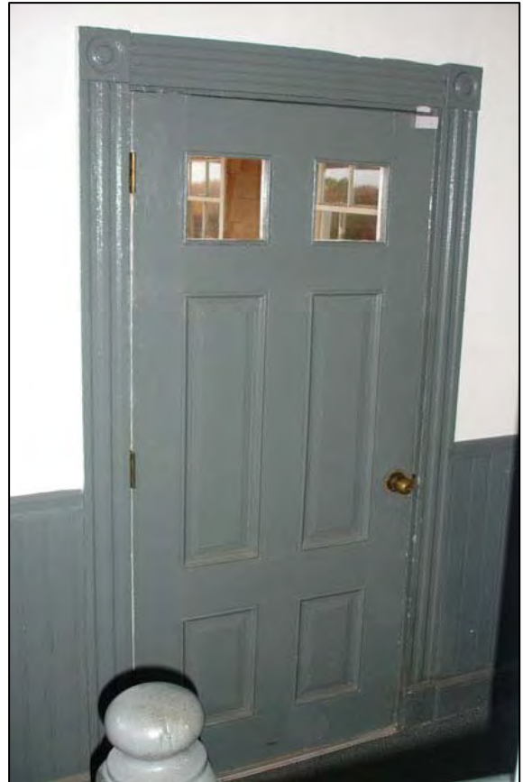
Figure 50. Spermaceti Cove Life-Saving Station, Room 101, D101.
