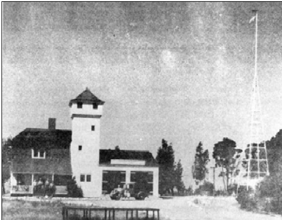
Figure 30. Spermaceti Cove Life-Saving Station, circa 1930, depicting east elevation exterior paint and steel tower north of station.
