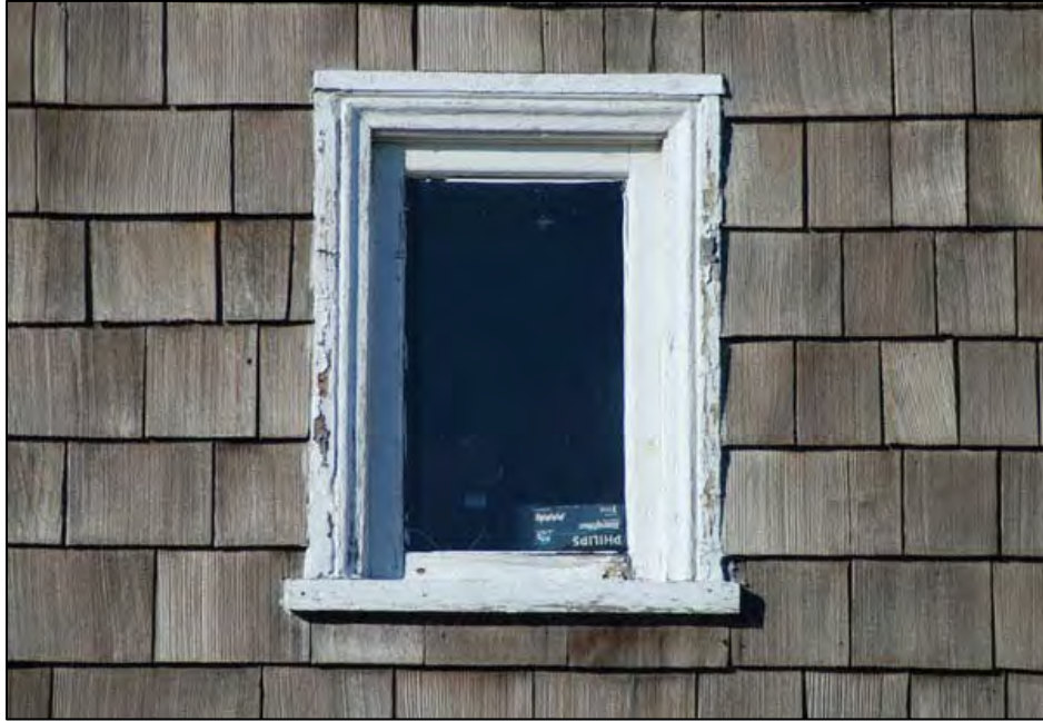
Figure 47. Spermaceti Cove Life-Saving Station, east elevation Tower window opening (W201) depicting historic molding.
