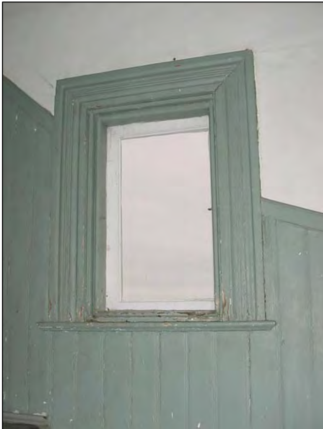
Figure 57. Spermaceti Cove Life-Saving Station, Room 201 W212 depicting window opening elements typical of Tower windows.
