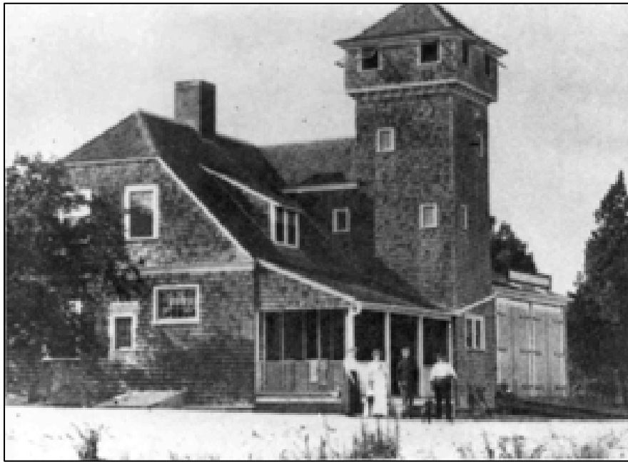
Figure 25. 1894 Spermaceti Cove Life-Saving Station circa 1910 after the basement was added and the Boat Room doors were altered.
