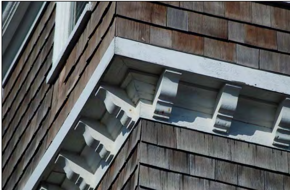
Figure 45. Spermaceti Cove Life-Saving Station, cornice below cantilevered section of Tower depicting brackets and molding.
