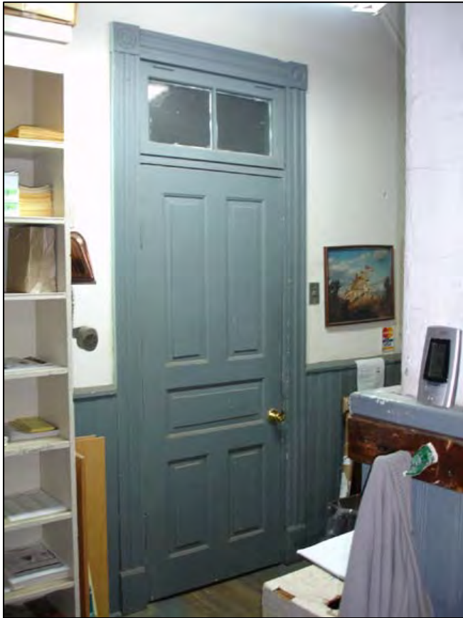
Figure 61. Spermaceti Cove Life-Saving Station, Room 206 D205.
