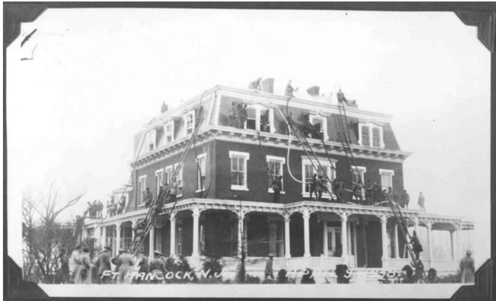
Fire at Fort Hancock Officers' Club, April 9, 1938.
