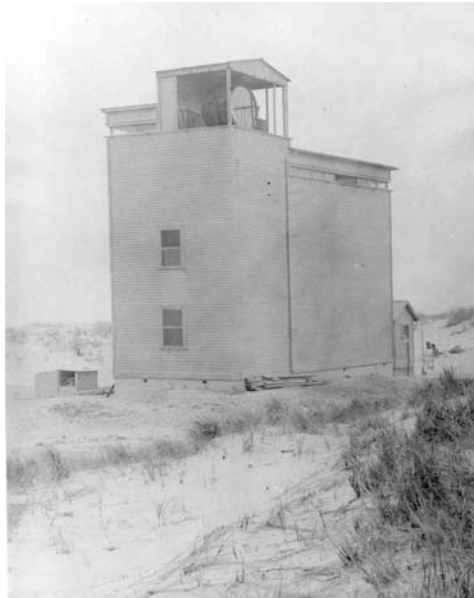
Coast Artillery Searchlight tower in wooden structure.
