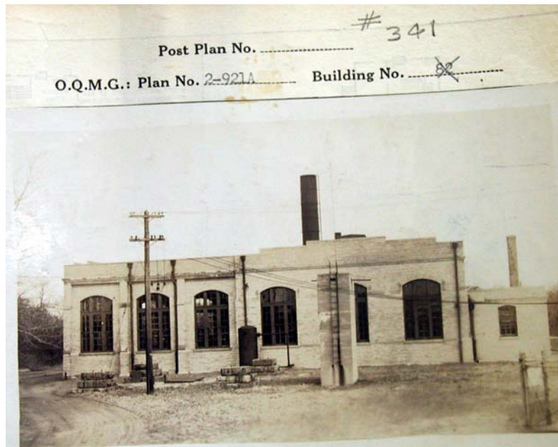
Fort Hancock Pumping Station
