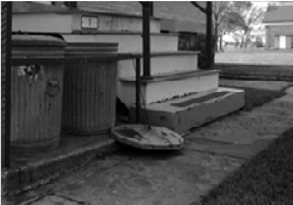
Figure 2.9. Some walkways surrounding the homes of Officers's Row are flagstone, like the one pictured above. Also note the trash can enclosures. OCLP, 2004.
