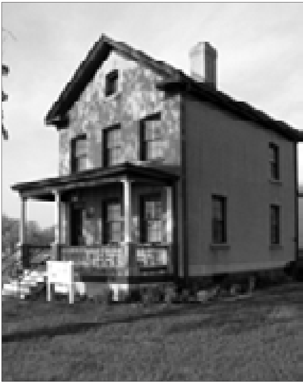
Figure 2.5. The building currently leased by the Audubon Society is typical of the smaller single family homes at Fort Hancock. OCLP, 2004.
