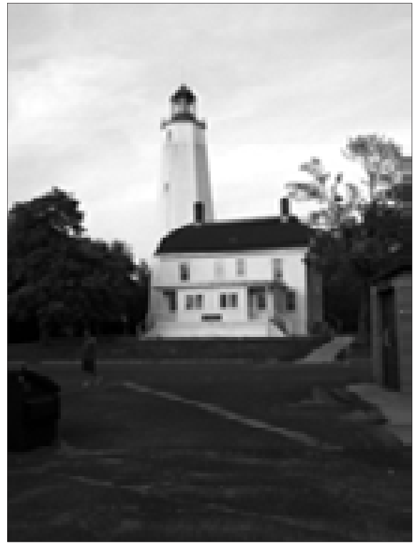
Figure 2.6. The Sandy Hook lighthouse and Keepers Quarters Museum. OCLP, 2004.
