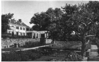
FIG. 87. HOUSE OF GEORGE B. AGNEW, ESQ., LEWISBORO, N. Y. William Adams, Architect.
