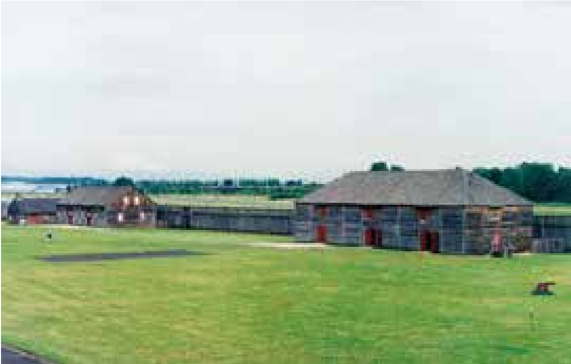
Asphalt pads within the palisade will be removed and historic building locations noted with corner markers. Additional reconstruction will occur within the fort palisade.
