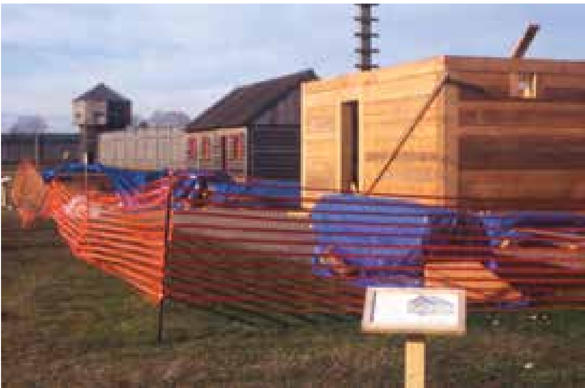
Recent reconstruction of the Jail within the fort palisade.
