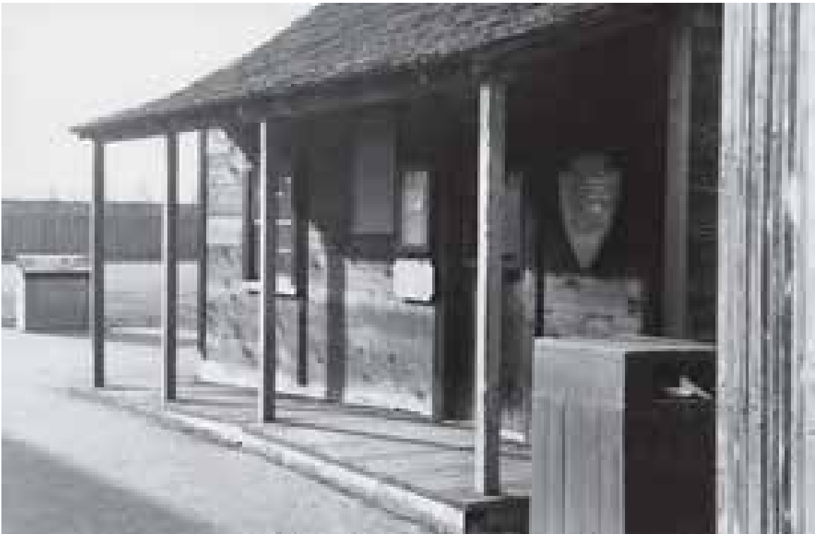
The non-historic contact station inside the fort palisade will be removed and eventually housed in a newly reconstructed Owyhee Church.
