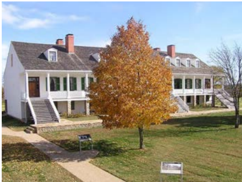
Figure 16. View of Officers' Row Quadrangle depicting Officers' Quarters HS-1 (left) and HS-2 (right). (PBA 2009)
