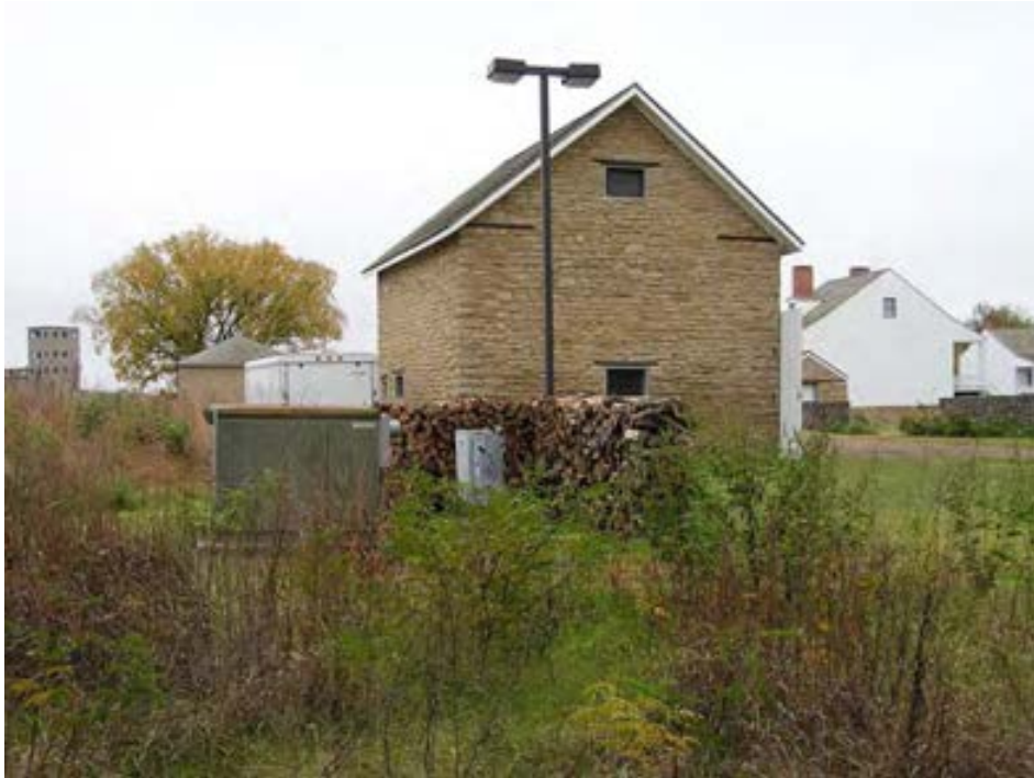
Figure 45. Wood piles used to minimize the visual intrusions of present day utilities such as mechanical units. (PBA 2009)
