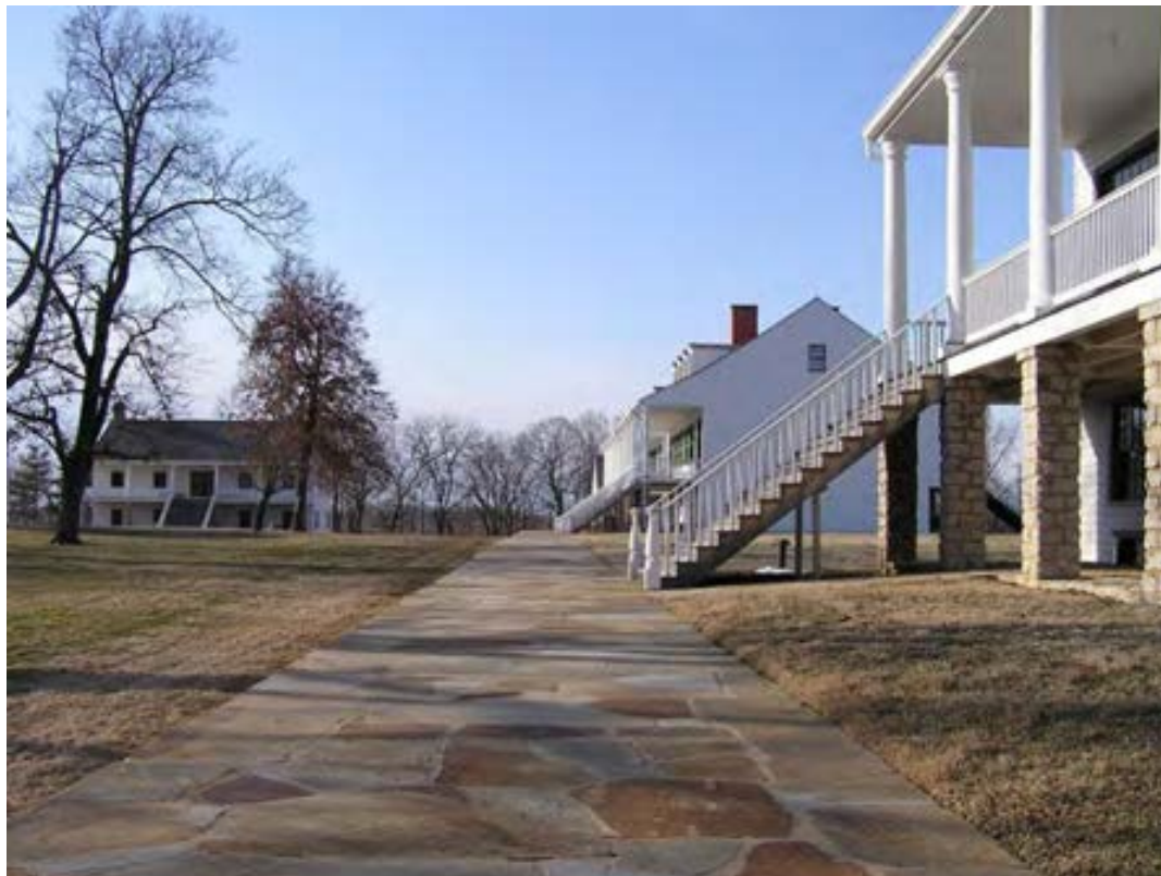
Figure 39. Flagstone walkway on the northeastern side of the Parade Ground that parallels Officers' Row. (PBA 2009)
