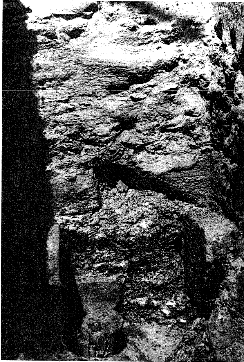
Illustration 11b Trench E - East Profile showing Fort foundations
