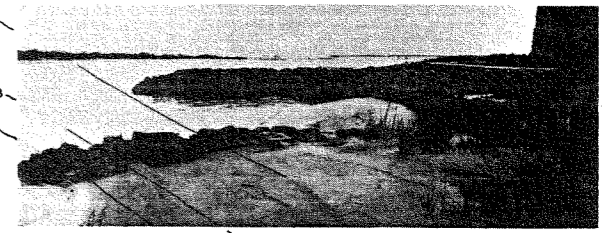
⑥ GROINS (#2 & 3), SEAWALL & 1937 BULKHEAD
