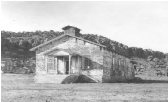
The post chapel at Fort Davis was a one-room school house.
