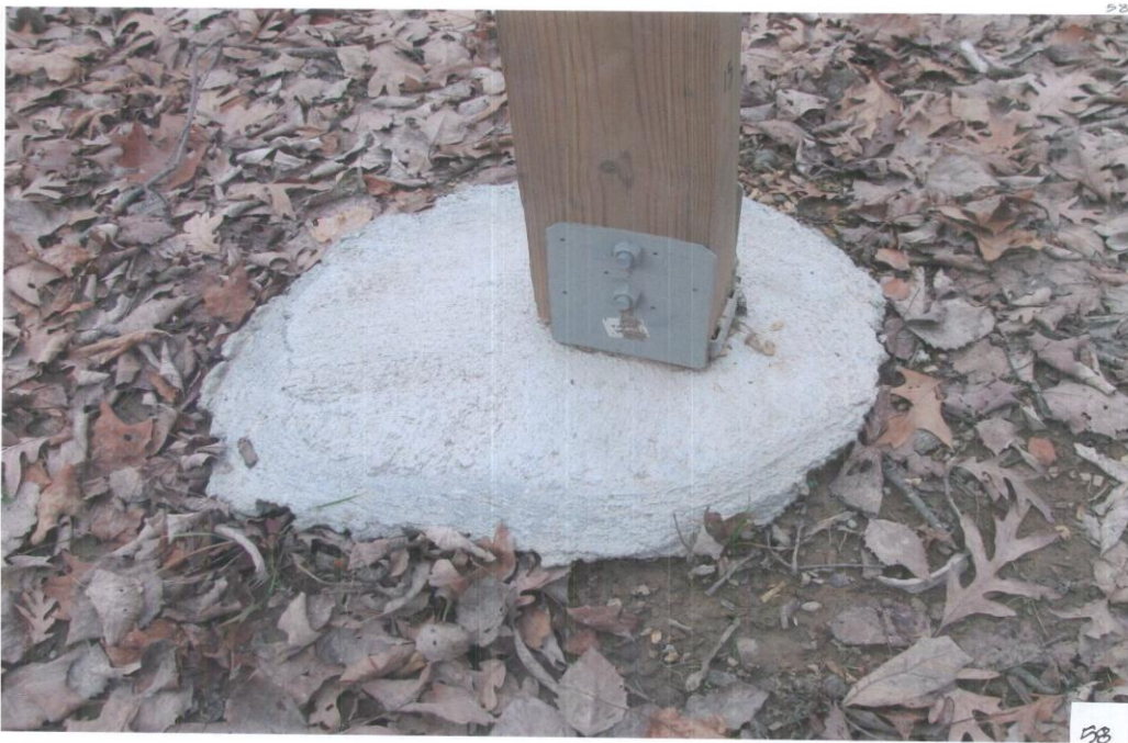
Figure 5. Detail of concrete post support.
