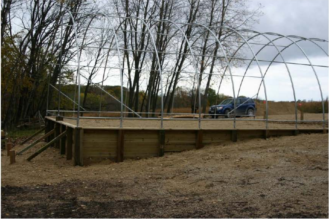
Figure __. Construction phase view of maintenance building.
