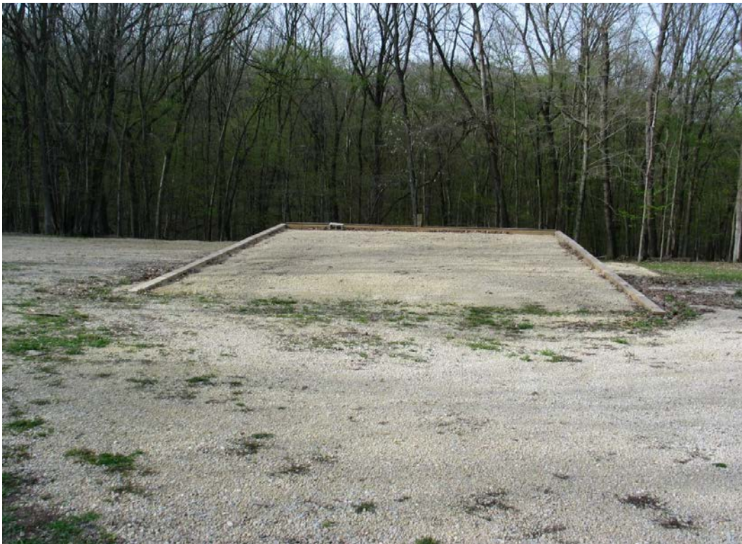
Figure 9. Maintenance building platform after construction and removal of superstructure.
