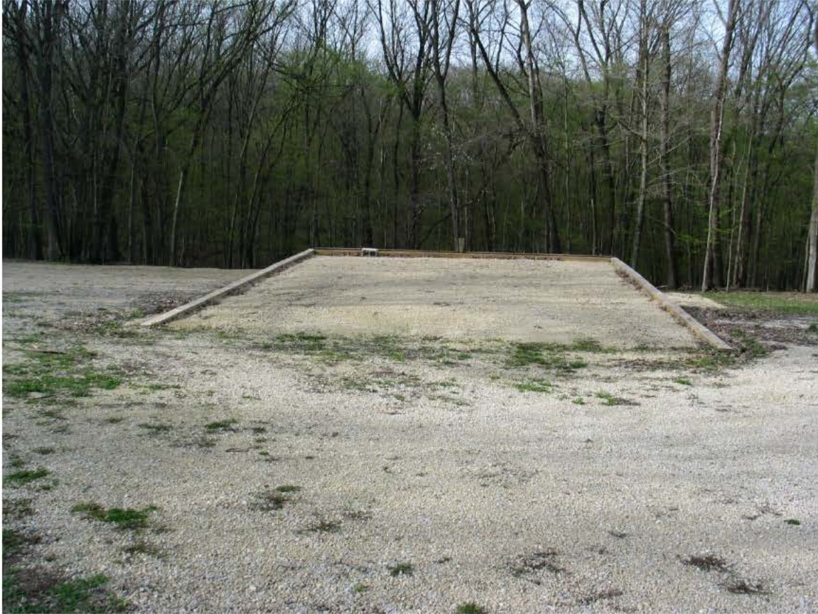
Figure . Maintenance building platform after construction and removal of superstructure.
