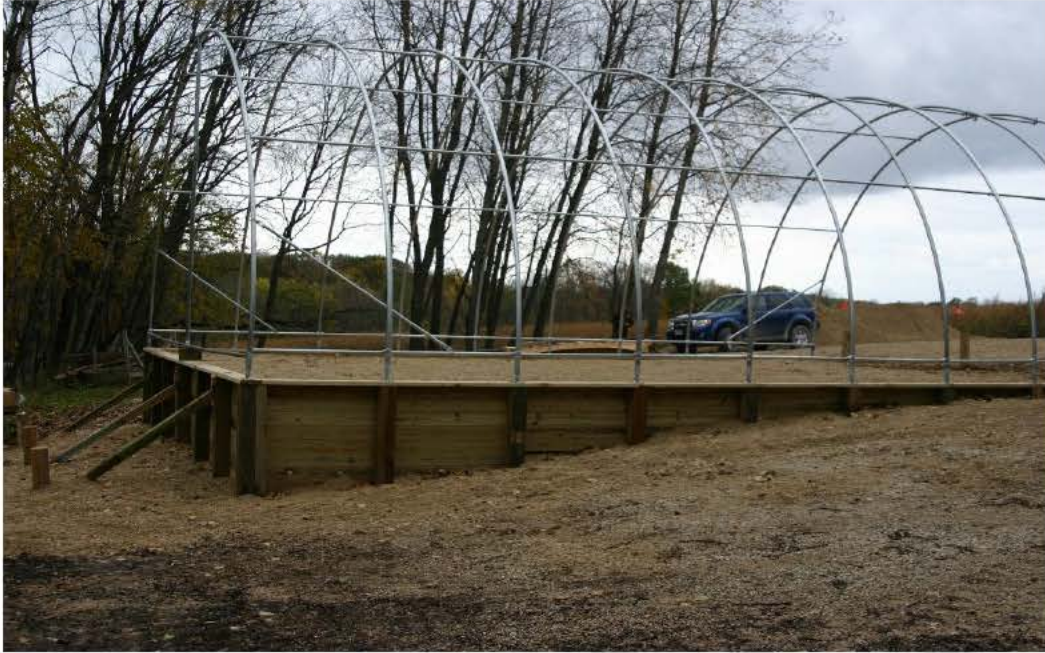
Figure 4. Construction phase view of maintenance building.
