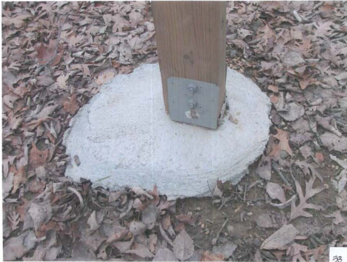
Figure . Detail of concrete post support.
