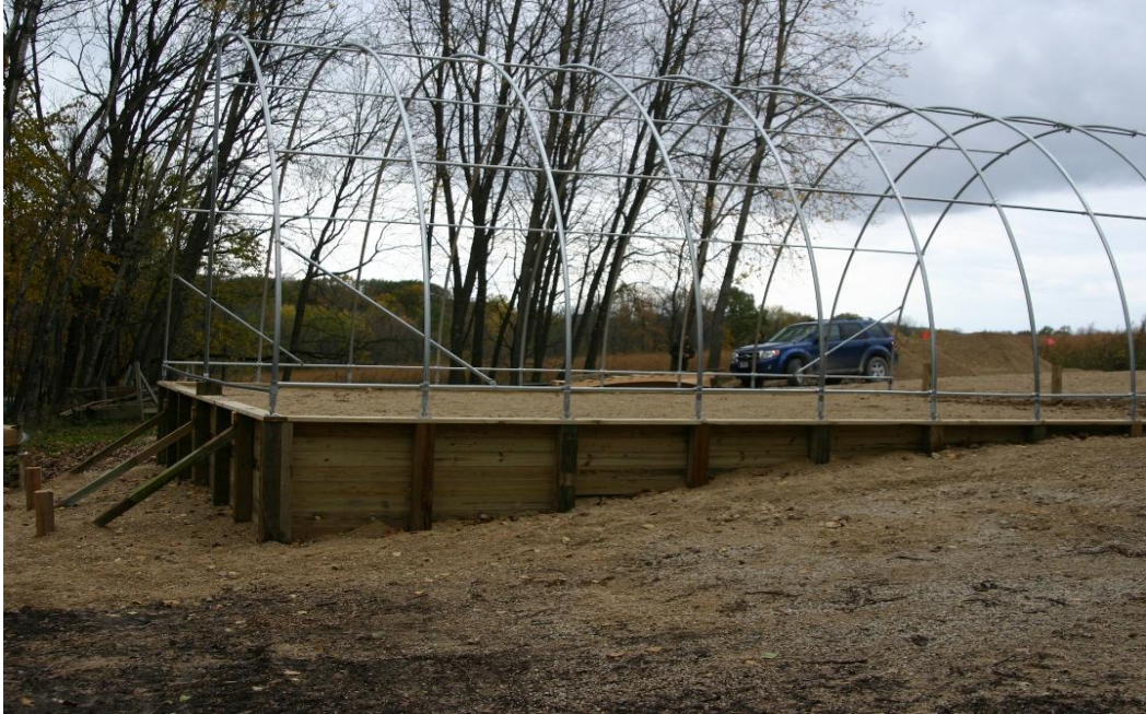
Figure 8. Construction phase view of maintenance building.
