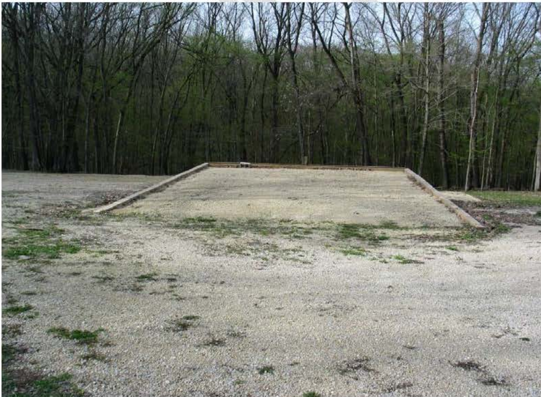
Figure 5. Maintenance building platform after construction and removal of superstructure.
