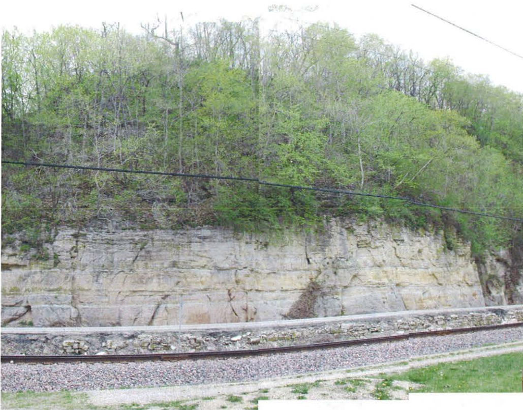
Figure 2. Example of area along the eastern boundary that was not inventoried due to safety hazards.
