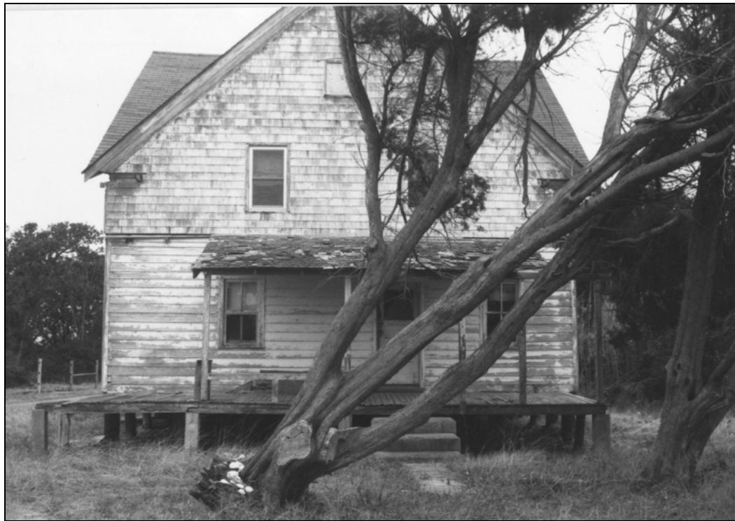
Figure 7.1.3. Abandoned House in Rodanthe. Photo by B. Garrity-Blake Photo.
