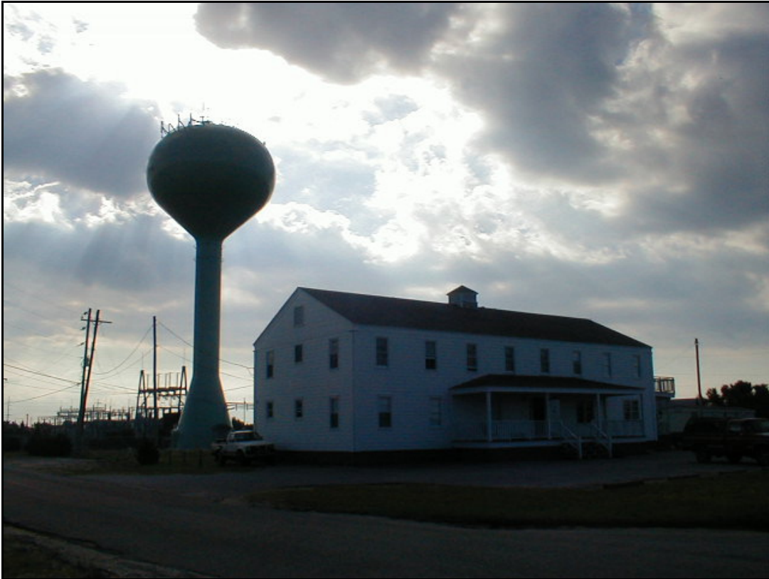
Figure 7.4.5. Old Avon Hotel next to Modern Water Tower. Photo by B. Garrity-Blake.
