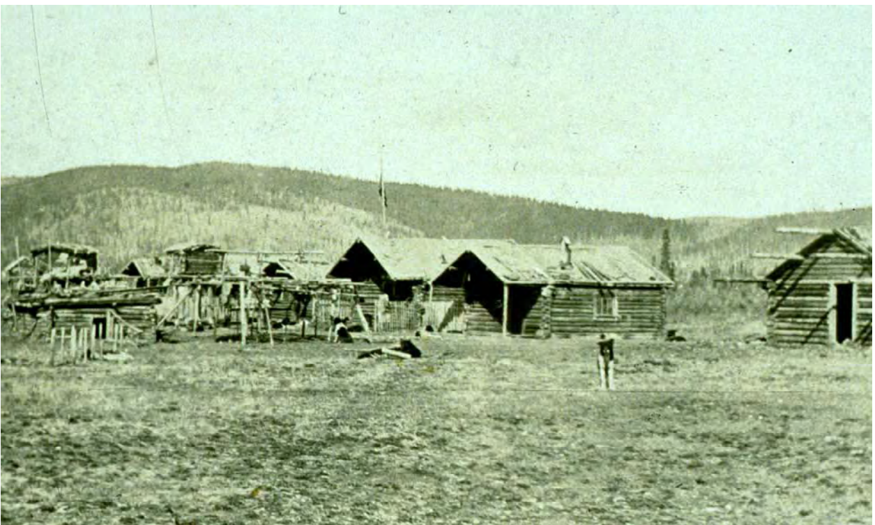
Plate 15. Tetlin in about 1919. By 1920 most Native people in the upper Tanana region were living in log cabins such as these. (Photo by F.B. Drane, courtesy of the University of Alaska).
