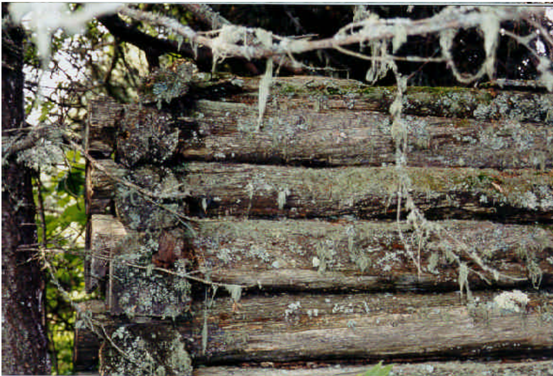
Figure 5.16 The remains of Hans' home today. Note the spruce tree growing against it (above) and the lichen and other deterioration accelerated by the shading (below).
