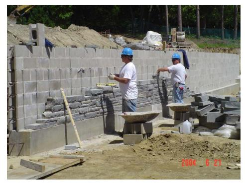
NHL mortar was used in this CMU retaining wall, as well as the stone veneer. Backfill heights were limited until the NHL mortar reached adequate strength.
