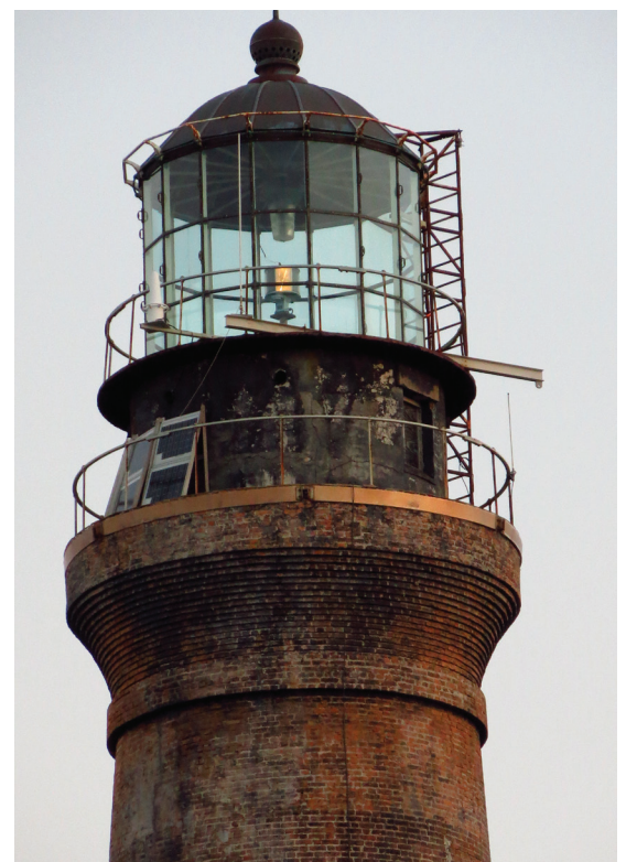
Loggerhead Lighthouse with Corbelled Masonry
