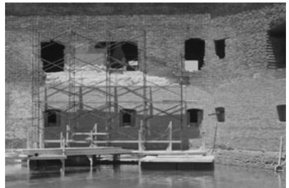
Ongoing work to stabilize Fort Jefferson's masonry.
