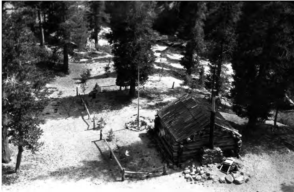
Overhead shot of the Postpile cabin. (From a 1936 NPS inspection report, Devils Postpile National Monument image collection)
