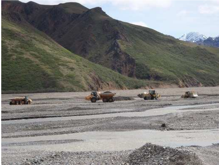
2012 Toklat “scrape”, i.e. gravel removal operation
