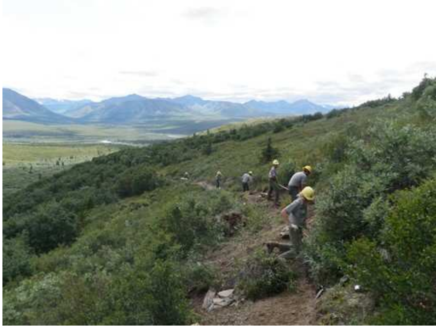
Trail crew working on Savage Alpine Trail
