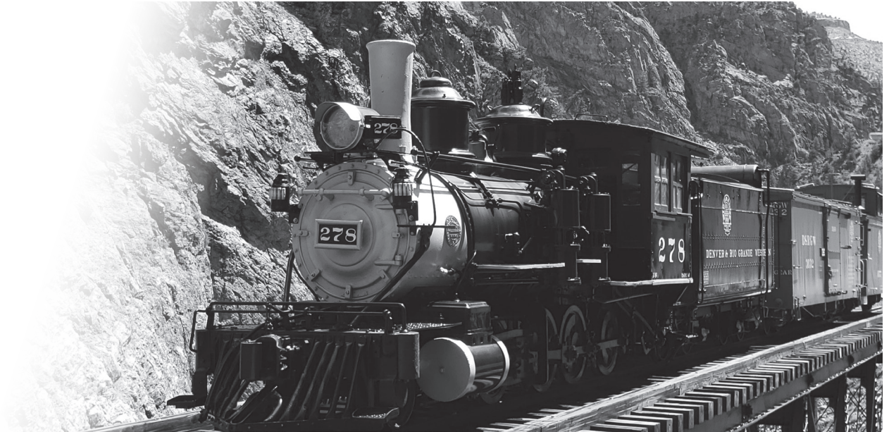
Engine #278 atop the truss bridge in Cimarron.
