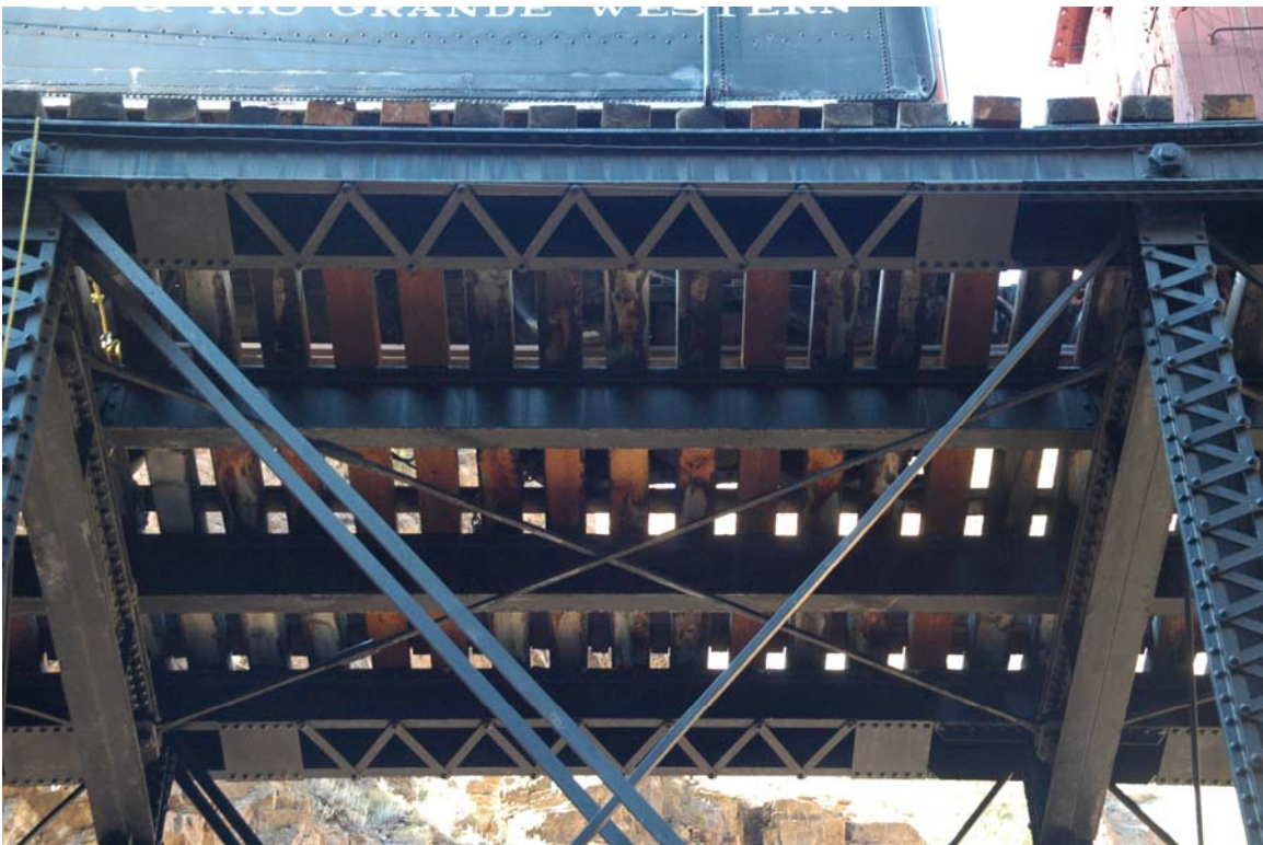
Figure 54. Under view of Truss
