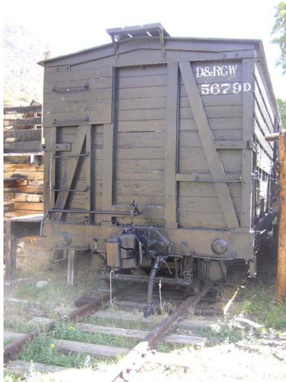
Figure 115. View of A end, Conditions of A, B end are good comparing to the other cars
