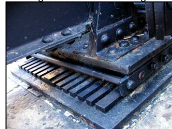
Figure 28: Roller bearings
