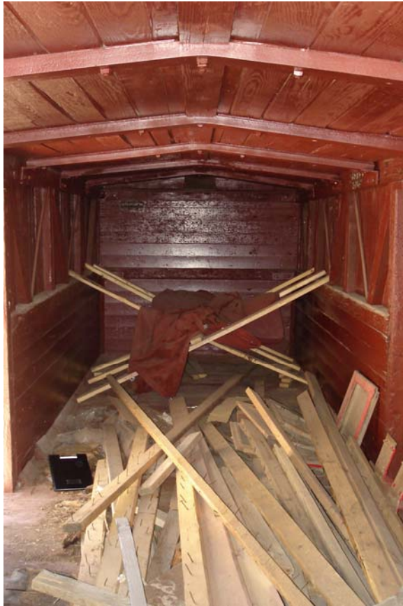
Figure 96. Inside view of B end under restoration work
