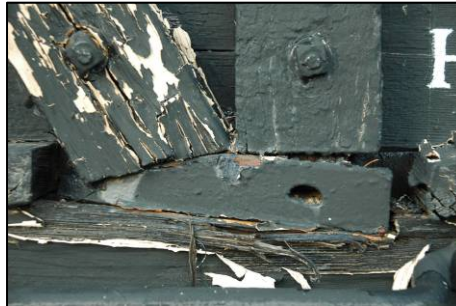
Figure 17: Left side angled wall post
