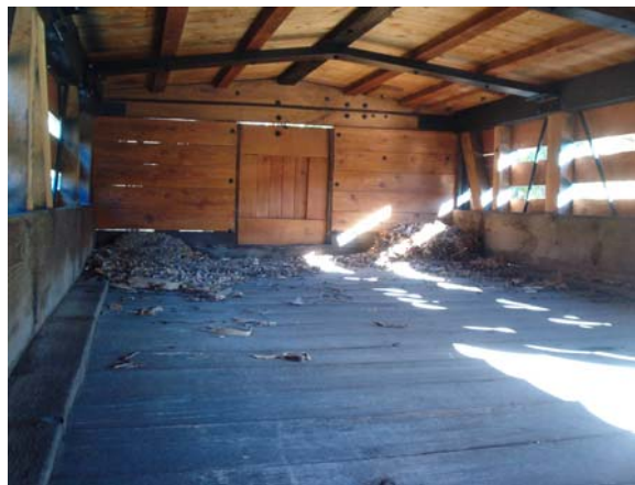
Figure 118. Inside view, newly changed material on the top and upper deck
