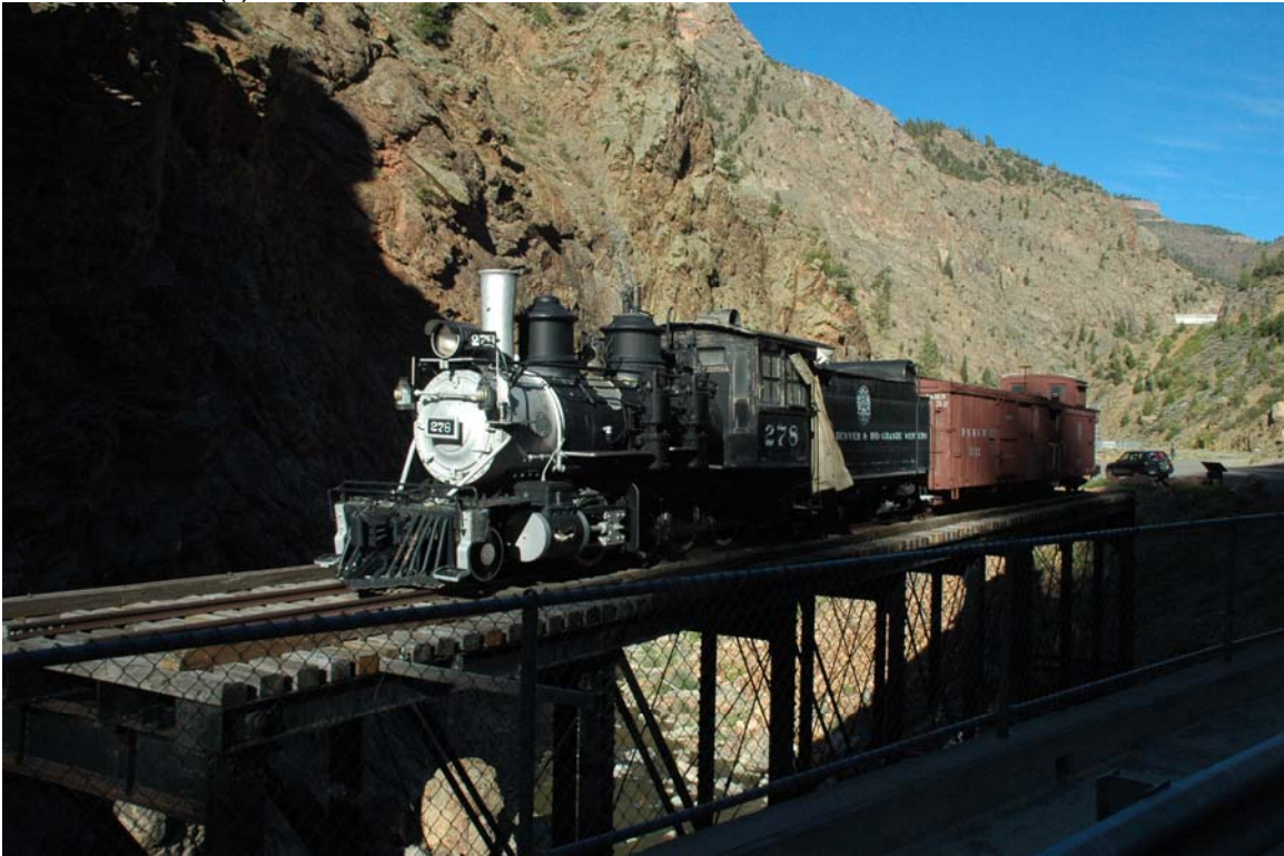
Figure 52. Overview of Locomotive on Truss
