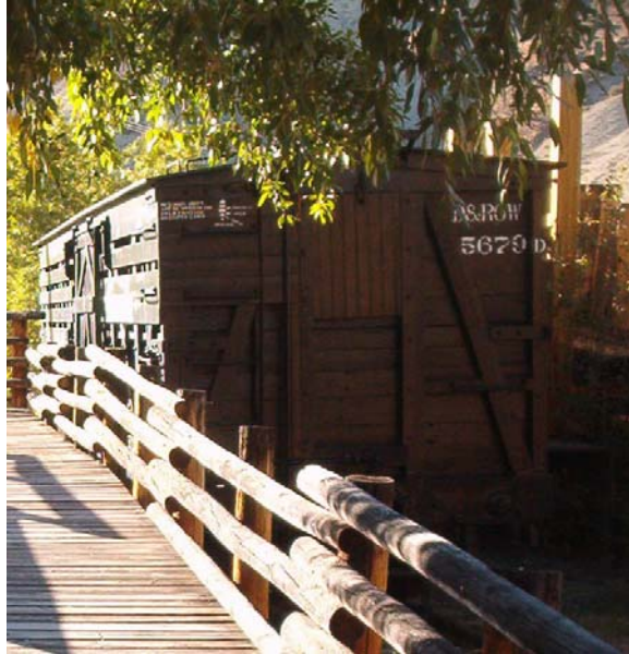
Figure 117. View of B end, A, B end are repaired recently
