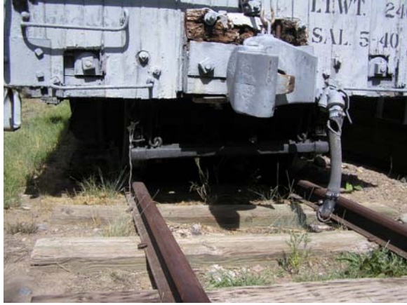
Figure 122. Rotten wooden part around coupler pocket of A end
