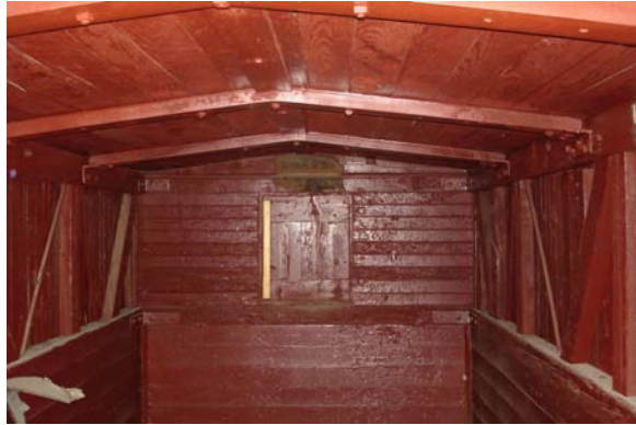
Figure 98. The inside of A end is newly repainted
