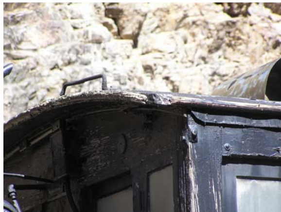
Figure 77. Weathered roof of engineer cab
