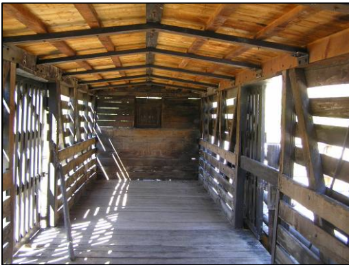
Figure 13: 5620 Interior looking A end to B end
