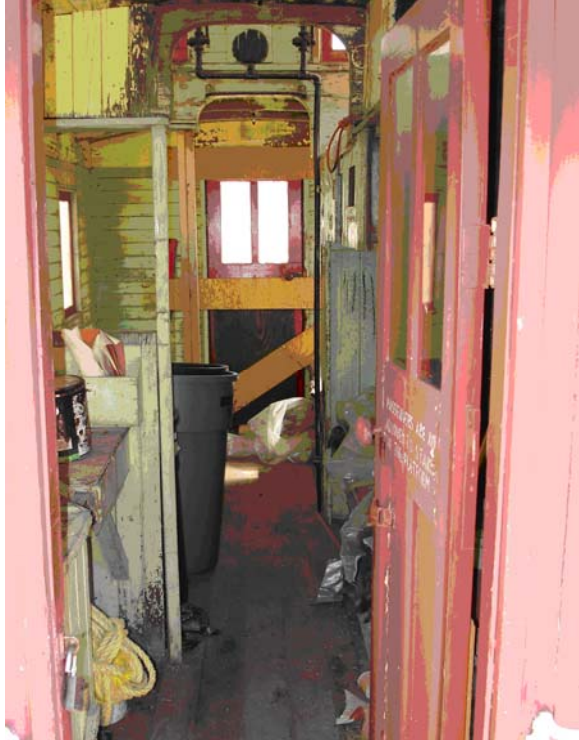
Figure 105. Debris and neglect accelerating deterioration
