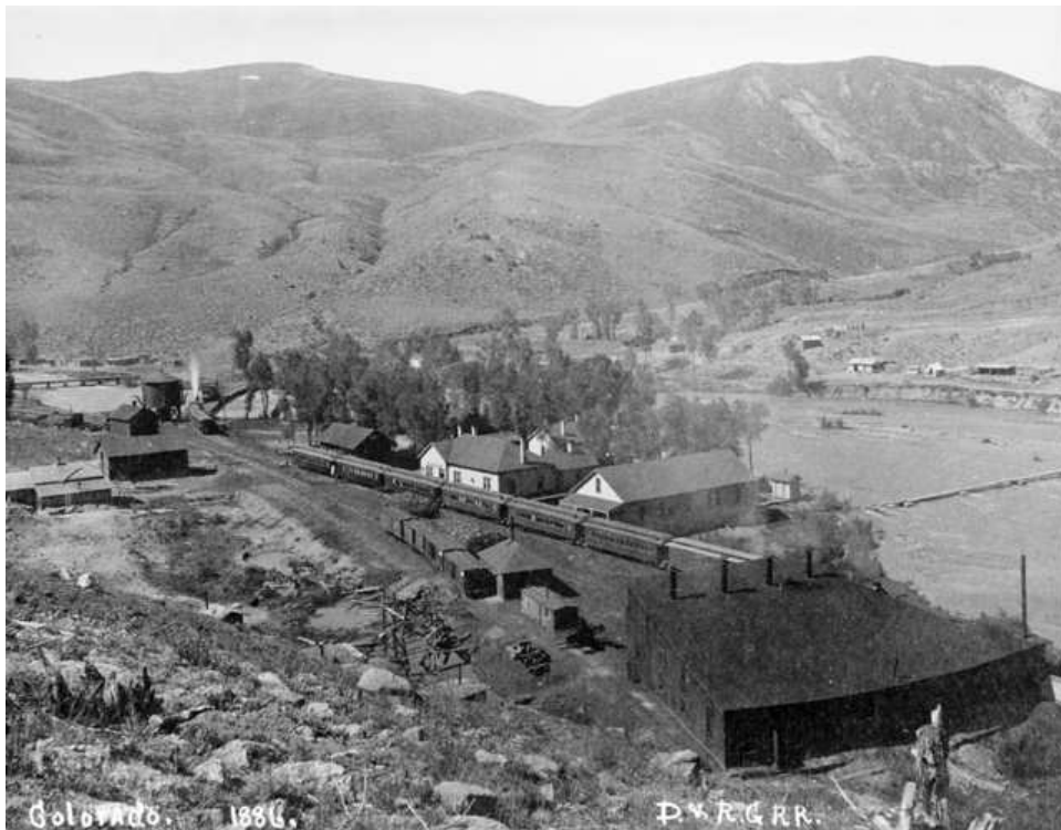
Figure 22. 1886 photograph of Cimarron – 1882 roundhouse in the foreground, Black Canon Hotel in the center, depot, and water tank – photograph by William Henry Jackson courtesy of Denver Public Library, Western History Collection
