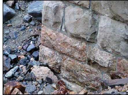
Figure 24: remnants of old granite pier
