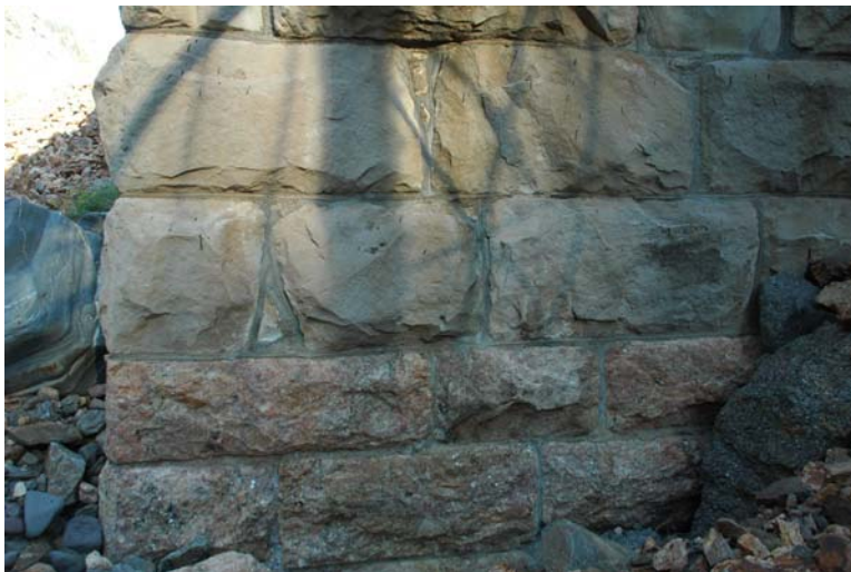
Figure 136. Newly repaired pier
