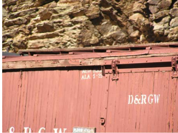
Figure 88. Paint on eaves moulding is peeling
