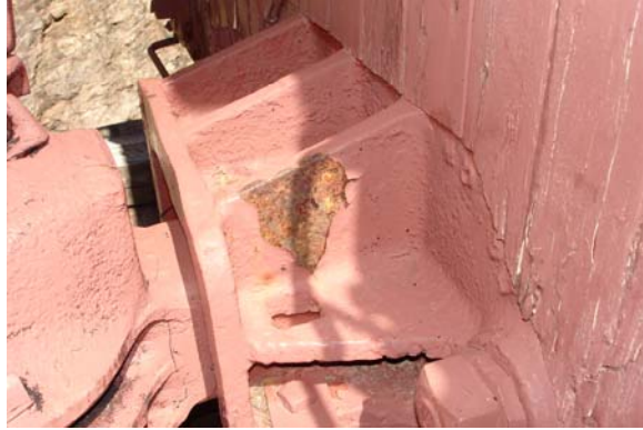
Figure 91. Rust and paint peeling on coupler pocket
