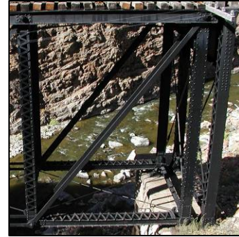
Figure 26: pin connections
