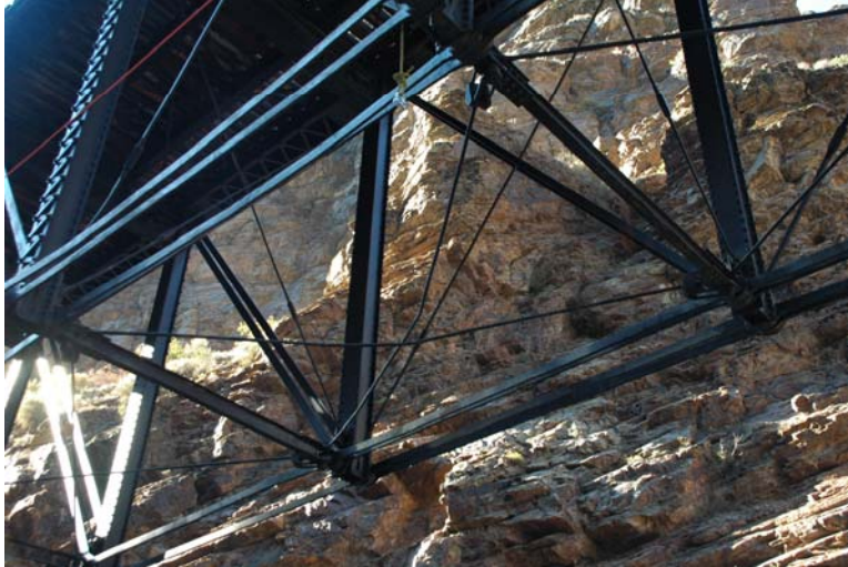
Figure 133. Diagonally bent cross tie bar
