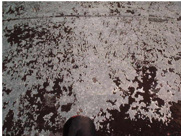
Figure 84. Roof top of engineer cab in bad condition
