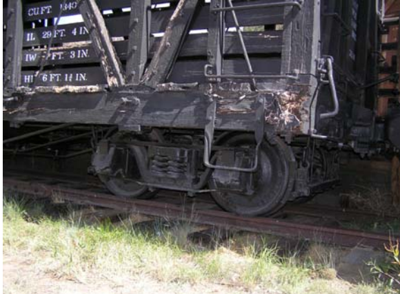
Figure 112. Undercarriage and rotten A end beam
