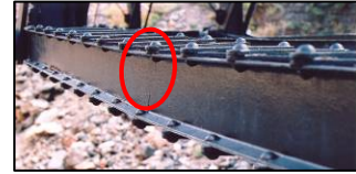
Figure 32: Cracked member
