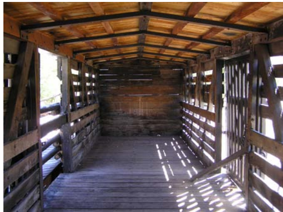
Figure 110. Inside view toward A end
