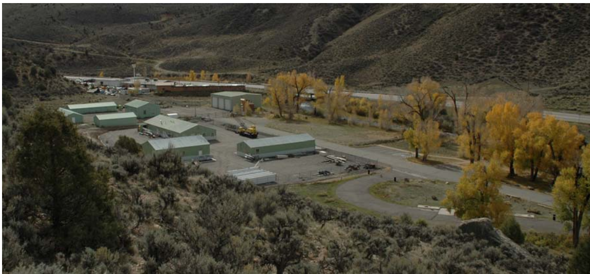
Figure 50. Maintenance facilities(Left) and RV dump(Right)
