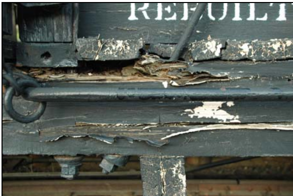
Figure 107. Right side B end rotten cross bar
