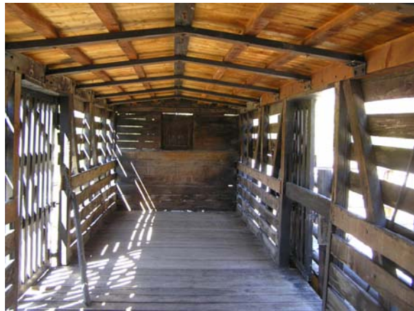
Figure 111. Inside view toward B end
