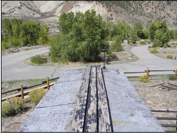
Figure 114. Roofwalk looking A end to B end
