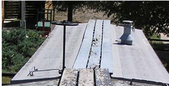
Figure 126. Roof view from B end to A end
