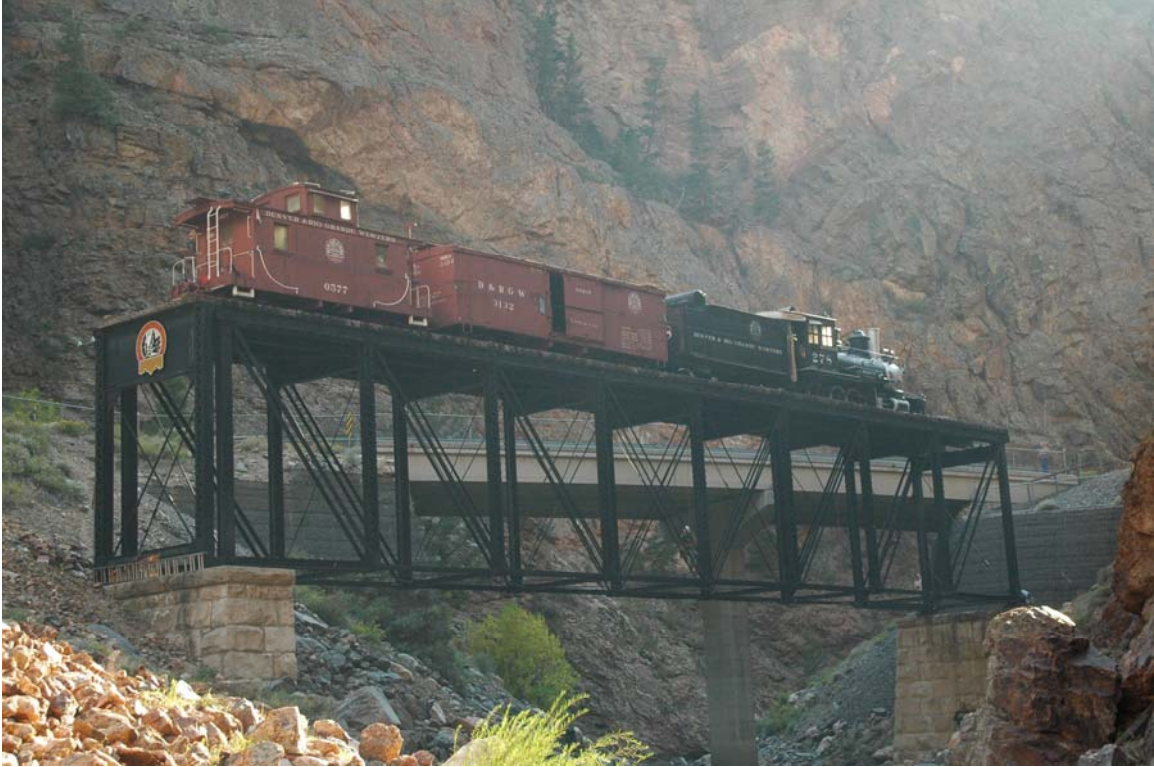
Figure 53. Overview of Truss
