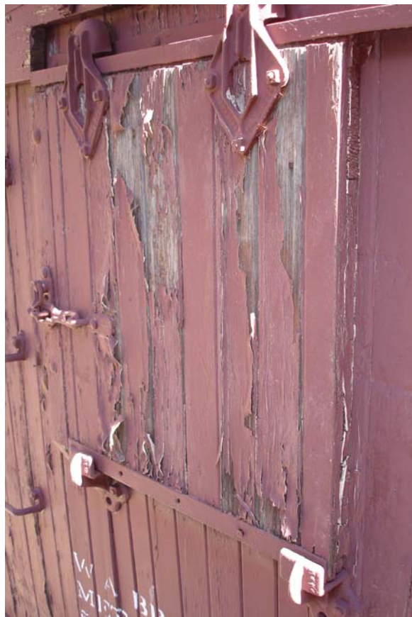
Figure 99. Paint is weathered
