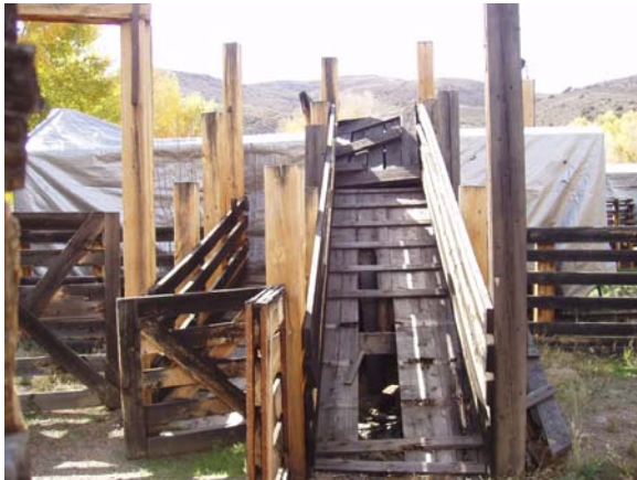
Figure 47. Loading deck for display
