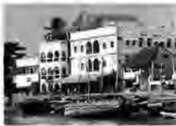
FIGURE 6 The well preserved Swahili town of Lamu on the Indian Ocean was the first gazetted historic district in Kenya and the first town to pass a local preservation ordinance. (Courtesy of the author)
