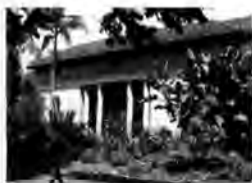
FIGURE 3 Headquartered in this building in Nairobi, the National Museums of Kenya is responsible for gazettement of Kenyan heritage under the Antiquities and Monuments Act. (Courtesy of the author)
