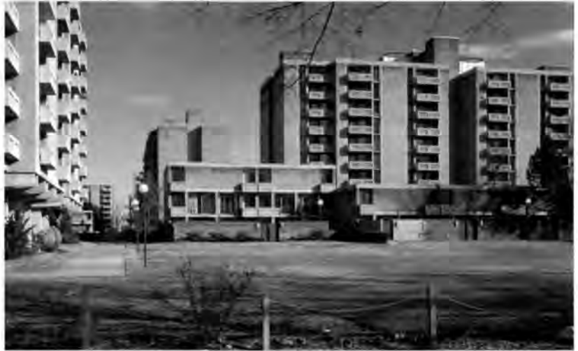
FIGURE 5 Tiber Island (1963-65) by Keyes, Condon & Lethbridge, shown in this view from 1991, was one of more than 10 housing projects that made Washington's Southwest Redevelopment Area one of the nation's most ambitious urban renewal undertakings. It was widely praised for the high caliber of its design. (Courtesy of the author)
