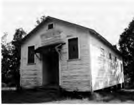
FIGURE 3 Constructed in 1926, the Bynum School in Panola County, MS, is typical of the modest construction of most Rosenwald Schools. (Courtesy of the Mississippi Department of Archives and History)
