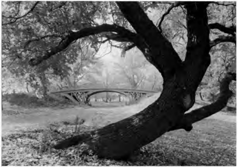
FIGURE 1 This 1984 photograph shows the cast iron bridge that spans the bridal path north of the reservoir in Central Park. (Photograph by Jet Lowe, courtesy of the Historic American Engineering Record Collection, Library of Congress)
