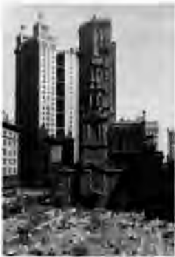
FIGURE 1 St. Paul's Chapel on Broadway in Lower Manhattan, shown here in a 1937 HABS photograph, has artistic, historic, spiritual, and economic value. (Photograph by Arnold Moses, courtesy of the Library of Congress)
