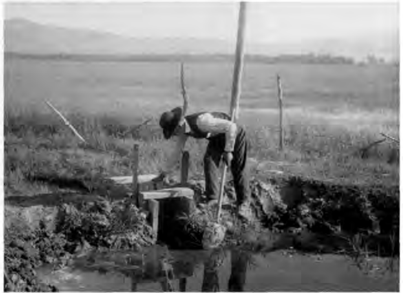
FIGURE 2 Photographed by Louis Charles McClure between 1908 and 1915, this view, entitled "Irrigation in Routt County," shows a simple wooden lateral turnout. (Courtesy of the Denver Public Library Western History Collection)
