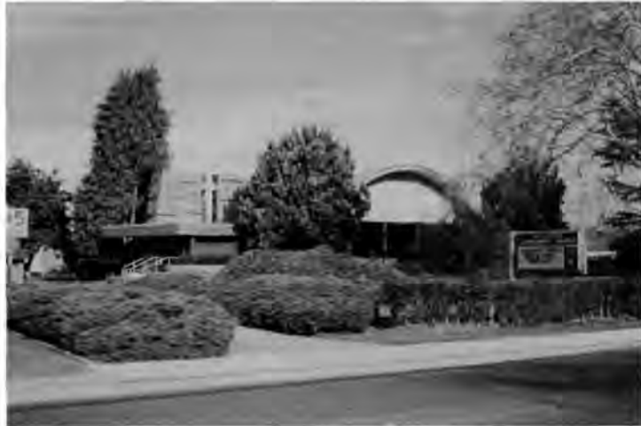
FIGURE 6 The San Lorenzo Community Church was constructed in the late 1940s from a World War II surplus Quonset Hut. (Courtesy of the author)
