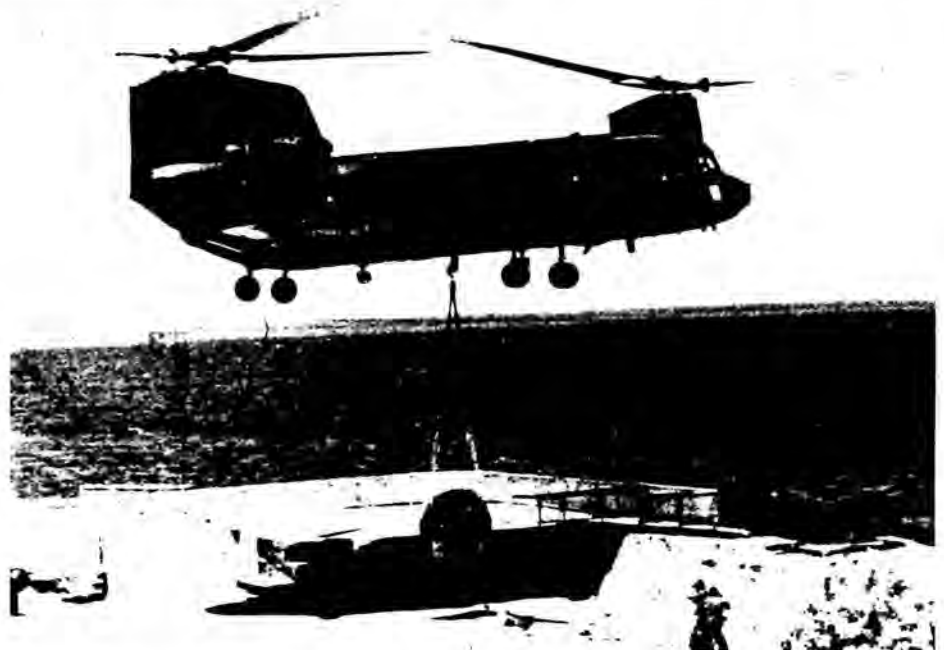
Base pivot mechanism being airlifted from the lower deck of El Morro.
