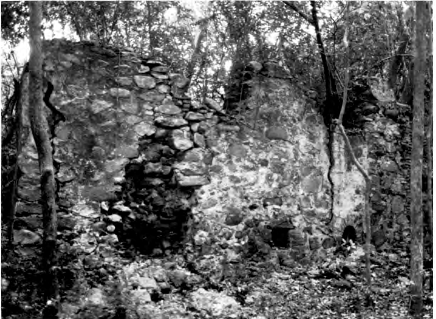
Exterior wall of the sugar boiling house at Plantation Zufriedenheit. The firebox for the Jamaica train is on the left end and vent openings are along the bottom of the wall. At the far right end of the wall are yellow brick traces of the former chimney for the boiling house.
