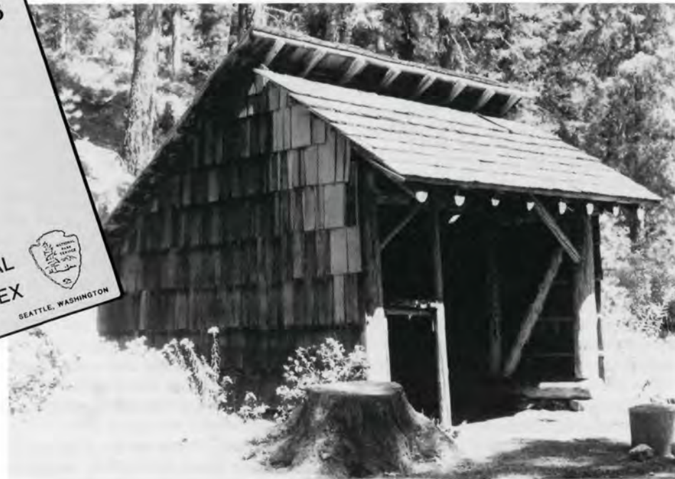
High Bridge Shelter, Lake Chelan National Recreation Area
