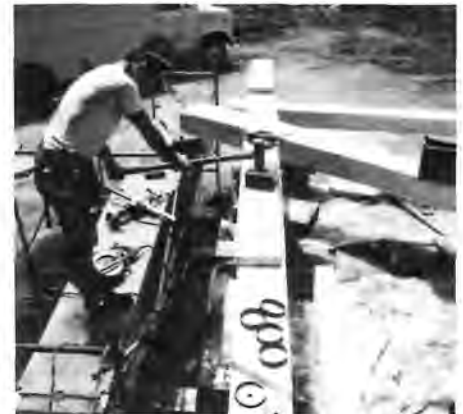
Shear connector rings.
