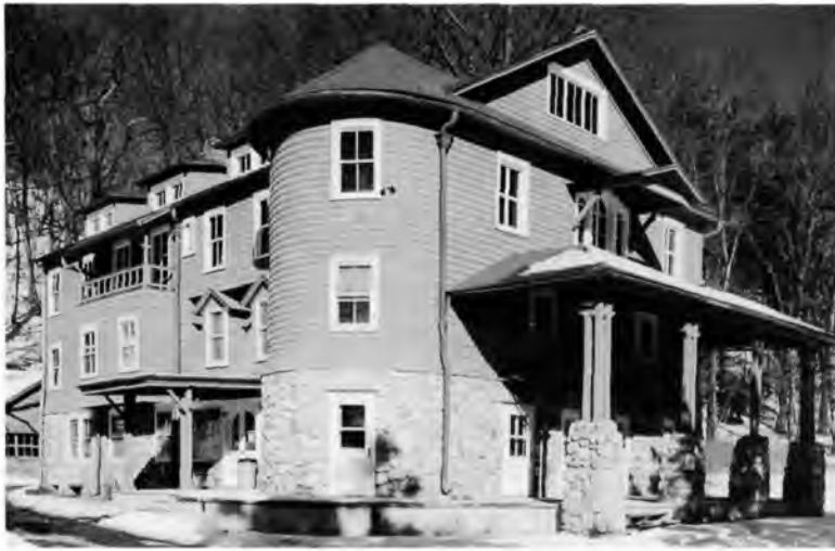
Arisbe, former home of American philosopher Charles S. Peirce, built c. 1887-1914.
