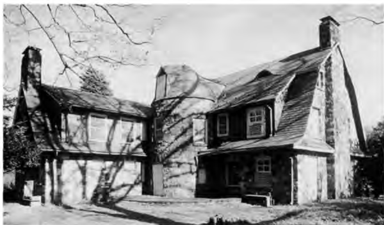
Zimmermann House, Dingmans Ferry, PA, built 1911, currently undergoing rehabilitation.
