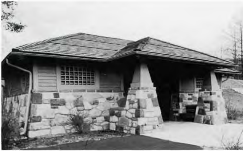
Restroom at Watergate Recreation Site, near Millbrook, NJ. The stone pattern of the foundation recalls the 1950s stone pillars of the adjacent dam that forms multi-level ponds. NPS photo.
