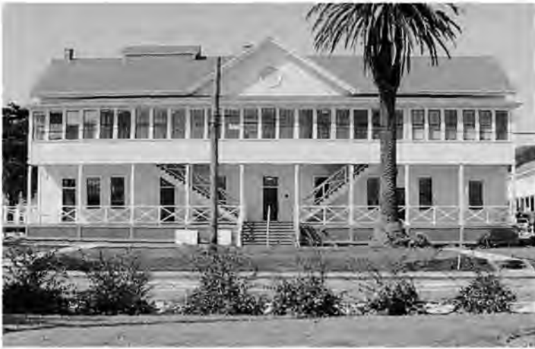
Building 36 after rehabilitation. Photo by Robert Wallace.
