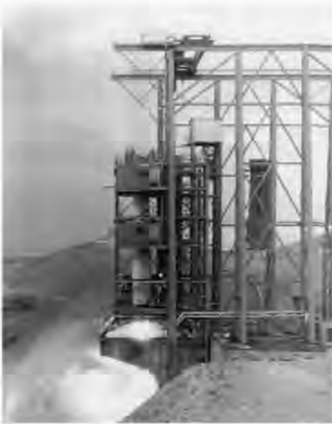
A propellant static test in progress on a major propellant test stand at Edwards AFB, 1958. Many of these Cold War-era structures remaining at Edwards AFB have been determined eligible for the National Register and were included in an inventory of California historic military buildings and structures funded by the Legacy program. Photo courtesy National Archives.
