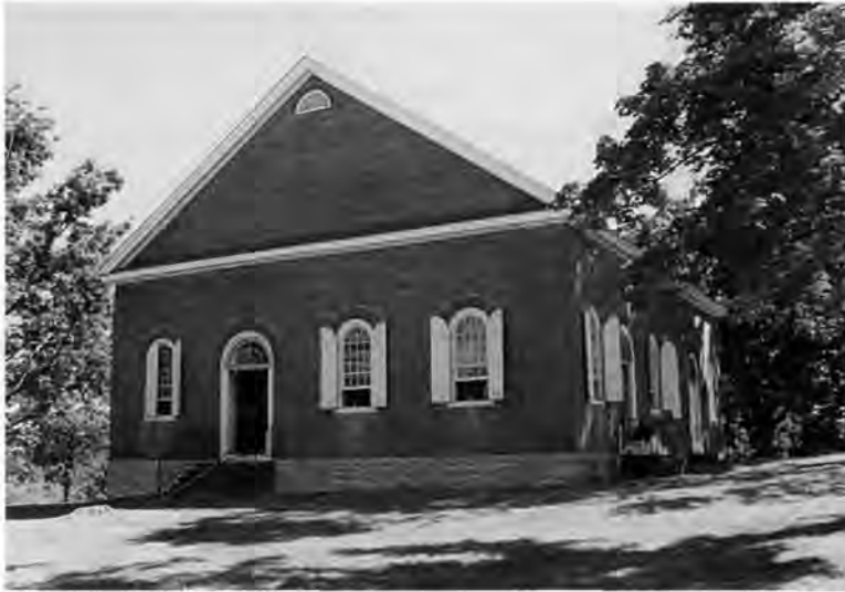
The 1794 Rocky Spring Presbyterian church with the original bricks reset with a soft mortar, all the trim work restored, and the pent roof restored. Photo taken July 3, 1997.
