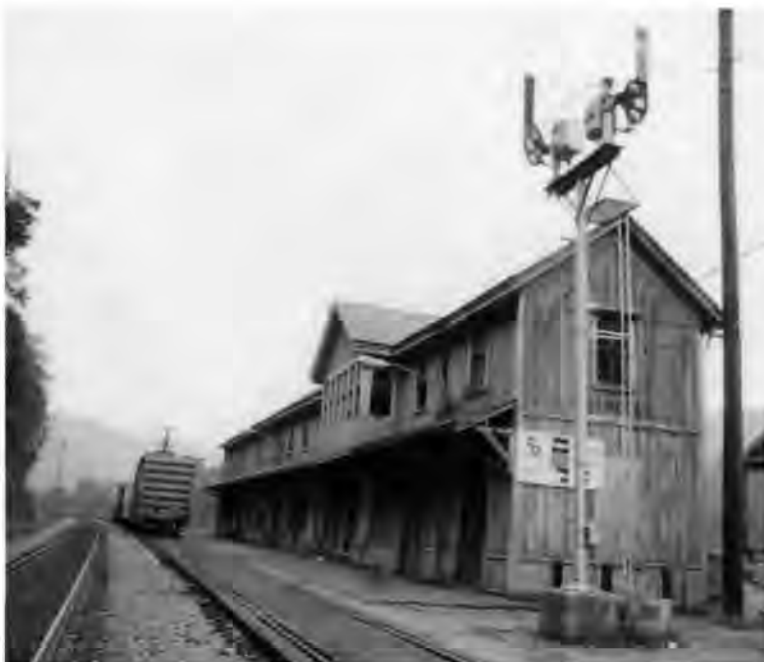
The 1904 Thurmond Depot of the Chesapeake and Ohio Railroad in the New River Gorge of West Virginia. HAER documented the site in 1988. IHTIA followed with historic structures and furnishings reports in 1992. Photo by Robert J. Hughes, 1990.
