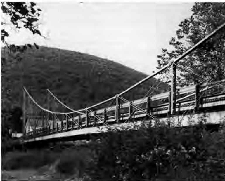
Lower Bridge at English Center, Pennsylvania, showing prominent catenary eye-bar chain and diagonal truss members. Photo by Joseph E. B. Elliott, 1997.
