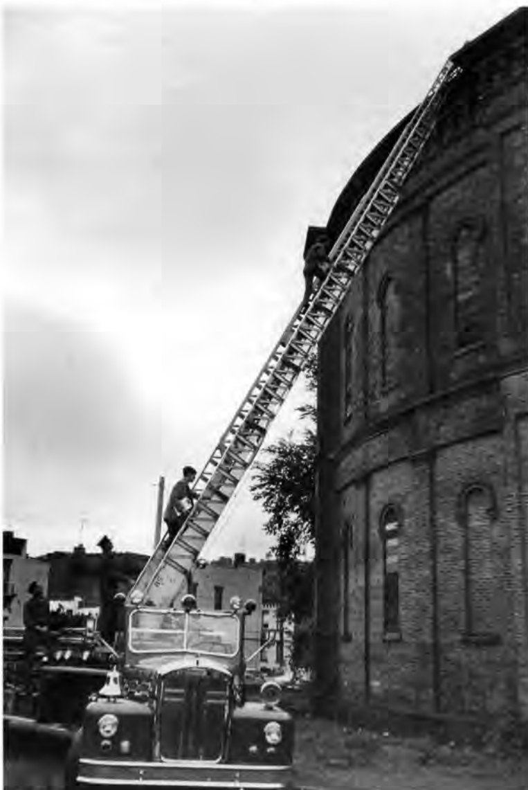
HAER team members David Bouse and Charles Parrott ascend a hook-and-ladder to measure the cornice of the Troy (NY) Gasholder house in 1969. Photo by Robert Vogel, 1969.
