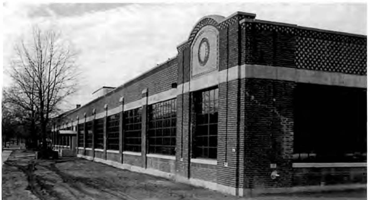
Building 661, former Machine Shop with reha- bilitation nearing completion, December 1999.
