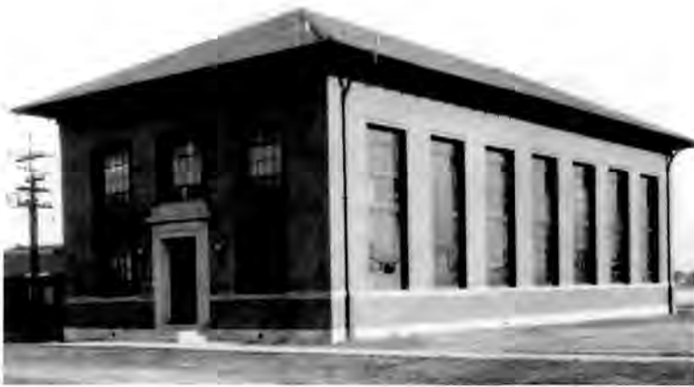
Building that housed the Atmospheric Wind Tunnel, the NACA's first wind tunnel (1920). Courtesy NASA Langley Research Center Photographic Archives.
