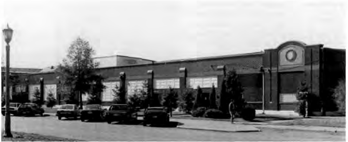
Building 661, former Machine Shop (c. 1995, before rehabili- tation).
