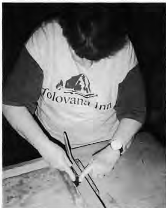
Marge Baldwin trimming off glazing compound at Midway recreation complex's game room.
