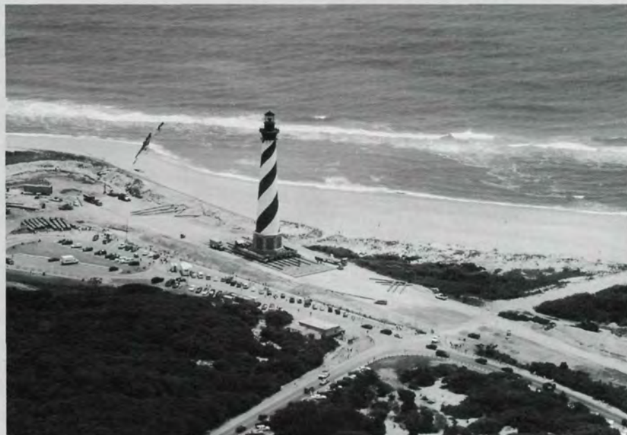
View of the move path of the Cape Hatteras Lighthouse.
