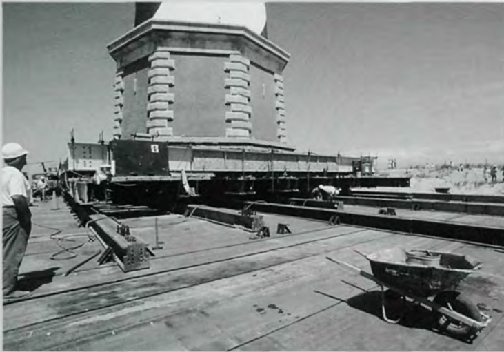
Above, the rail and steel mat are constantly moved forward. Right, the lighthouse about 600 feet from its original site.
