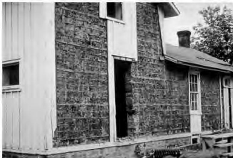
When it was demolished in the 1970s, this board-and-batten sided building in Geneva was found to be load bearing mud brick construction, originally sided with wood. Photo by David Brumberg.
