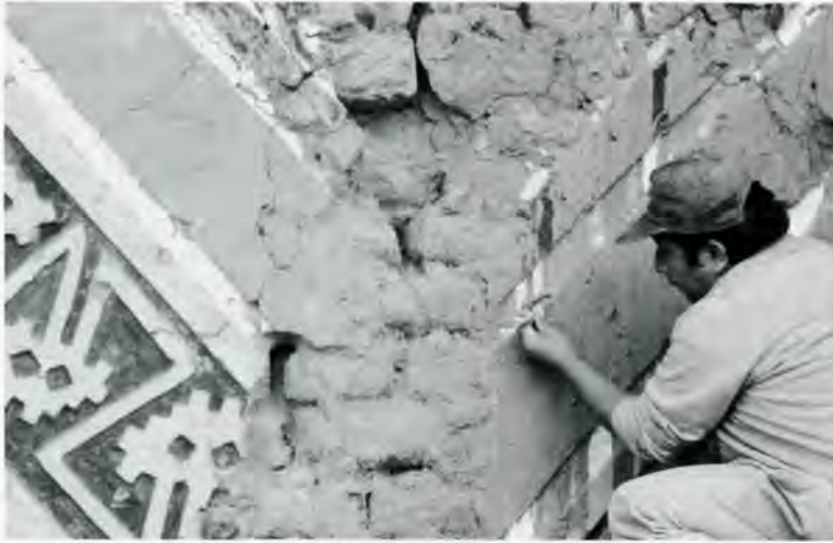
Huaca de la Luna, Trujillo, Perú. Cleaning and conservation of murals on recently excavated earthen architecture. Photo courtesy Michael Romero Taylor.
