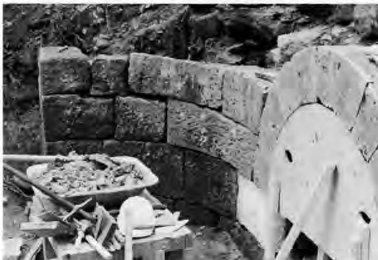
Dismantled culvert—backer wall exposed, culvert 1733.
