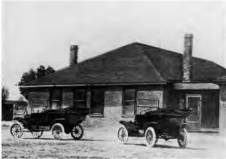
Campbell's Hotel in Adamana, Arizona served patrons of the Atchison, Topeka and Santa Fe Railroad. The proprietor was also custodian of the monument from 1912-1918.
