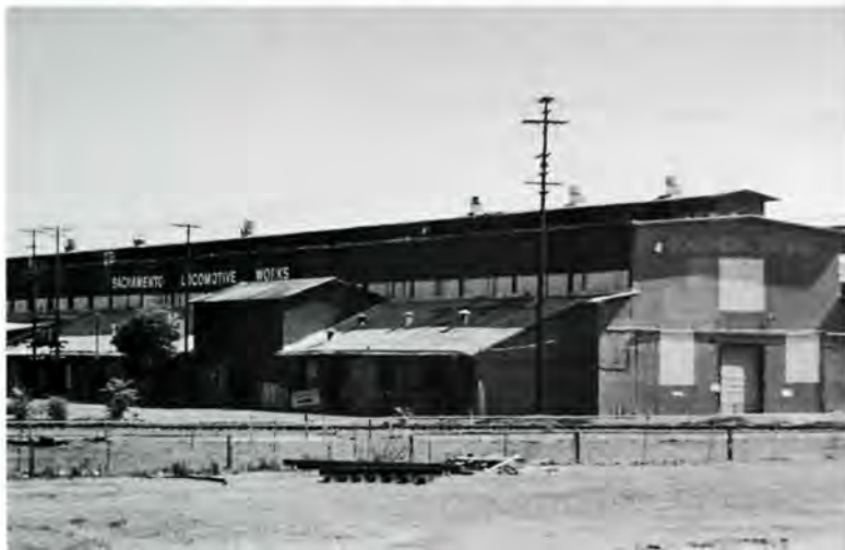
Sacramento Locomotive Works, showing boiler shop built c. 1888 with additions in 1905 and 1914.
