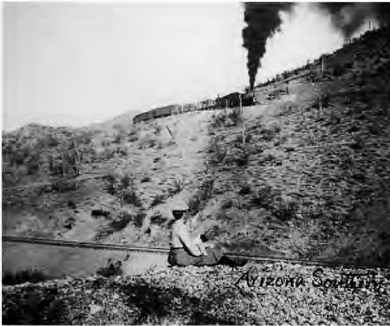
Unidentified woman and dog watching Arizona Southern coming into town, 1907. Train is moving forward on the middle switchback on Jesuit Hill just prior to backing into town on the upper switchback. Courtesy Special Collections Division, University of Arizona Library, Tucson, William F. Staunton collection.
