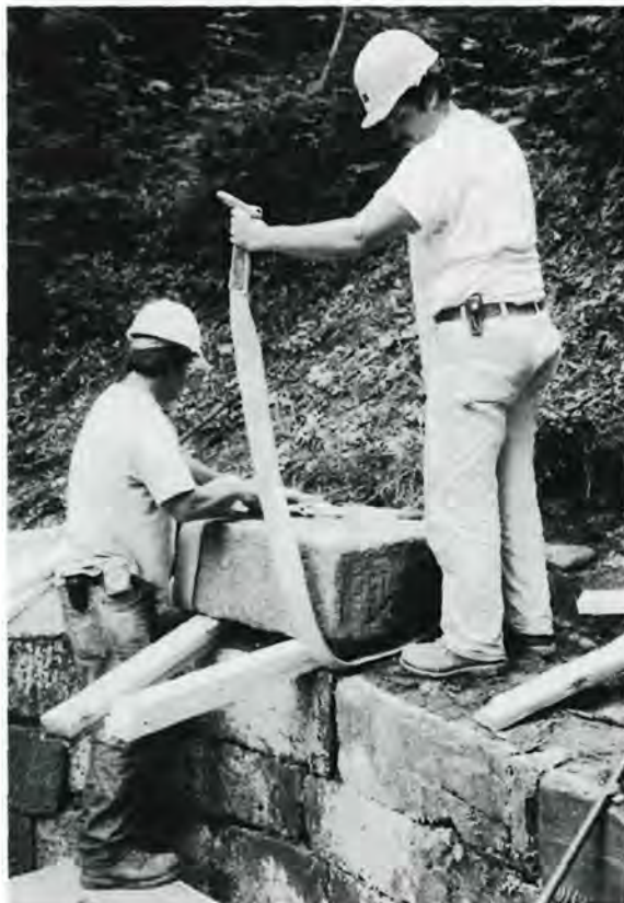
Dismantling process—coping course, culvert 1733.
