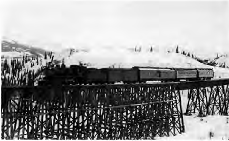
Riley Creek Trestle spans one of the two most difficult gorges to be bridged by the AEC. Photo by Grant Pearson, 1933-1934, courtesy Denali National Park and Preserve.
