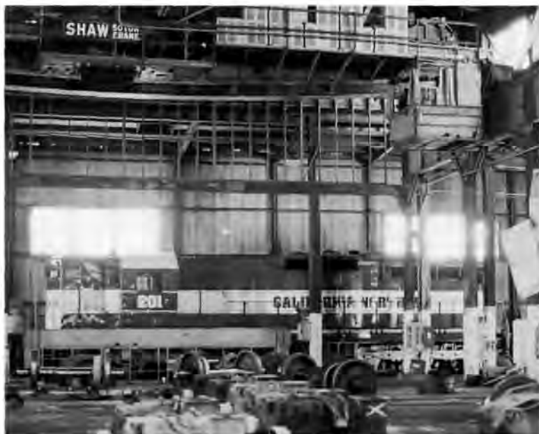
Sacramento General Shops, Southern Pacific Railroad. Interior of locomotive machine/erecting shop. Note California Northern Diesel-electric locomotive no. 201.
