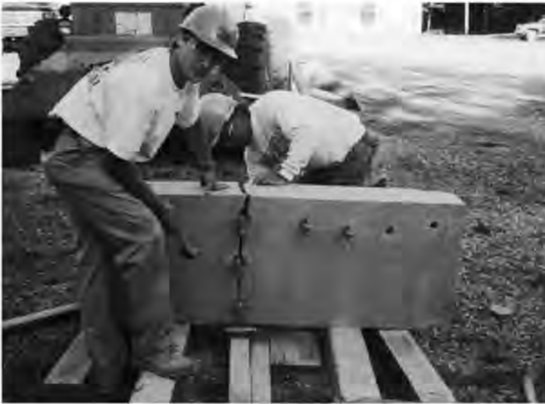
Splitting sandstone slabs for culvert 1656 using feathers and wedges.
