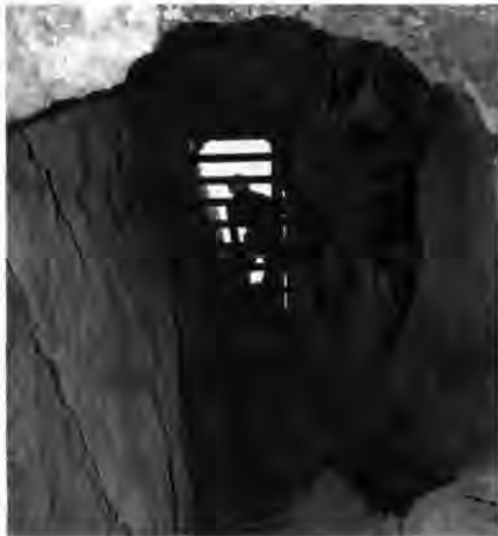
A bat-compatible closure or "bat gate" at one of the adit entrances of an abandoned manganese mine in New Mexico. The gate blocks human entry but lets the three species of bats that use the mine come and go freely.
