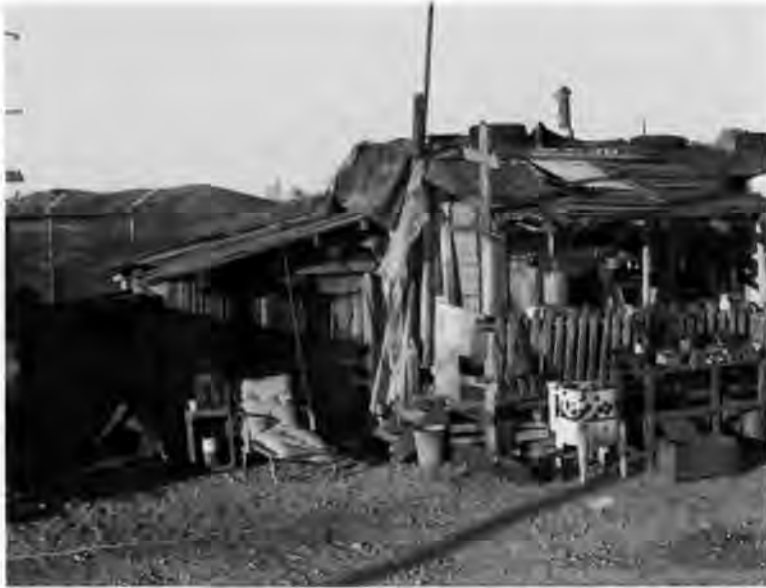
Designed and fabricated "historic residence" for filming of The Brave .
