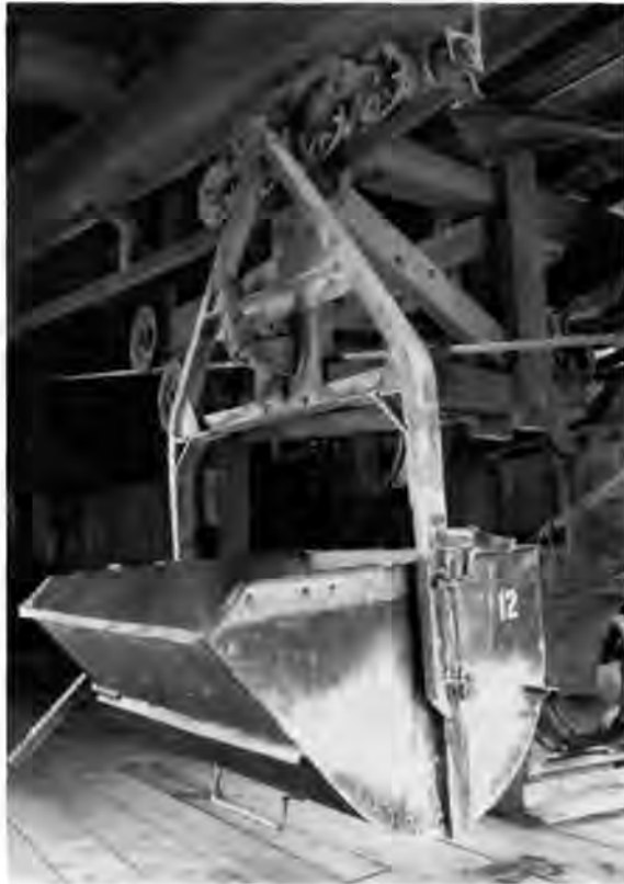
Ore bucket located within the tramway terminal at the Mayflower Mill.
