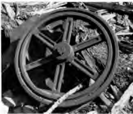
Collapsed Cracker Mill and bull wheel.
