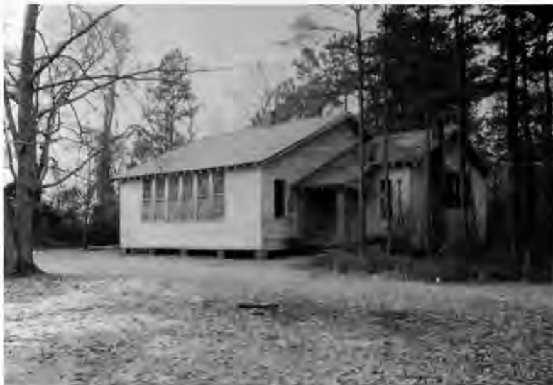
The St. Phillip School (1938) typifies the schoolhouses erected in rural South Carolina for African-American students prior to desegregation in the 1950s and 1960s. Photo by David G. Blick.
